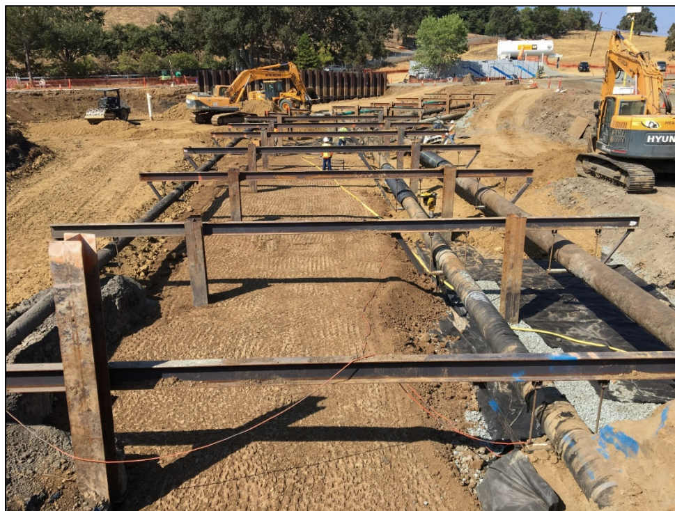
Figure 2. Cleanup excavation in progress – house demolished
