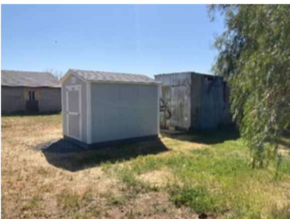
View of a new shed parallel with the well-head shed
