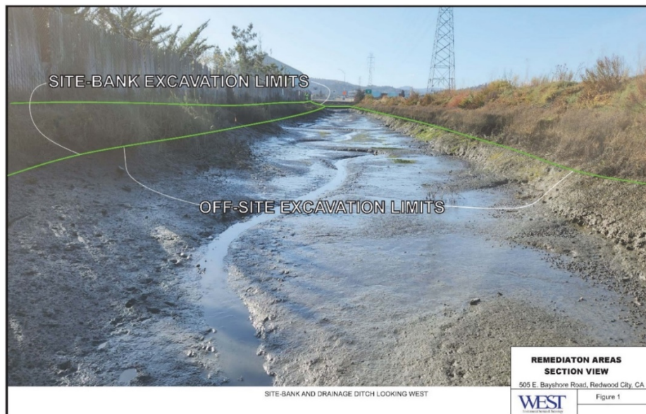
Figure 1: Photo showing the drainage ditch and excavation area of the off-site sediment.
