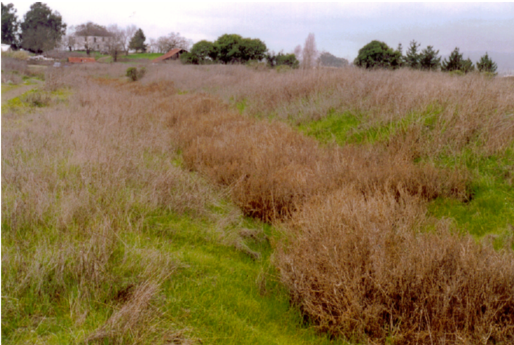
Drainage ditch DD 1 looking north
