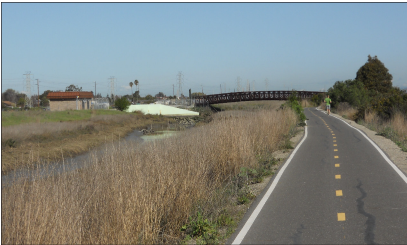
Viewpoint C: Middle reach looking downstream
