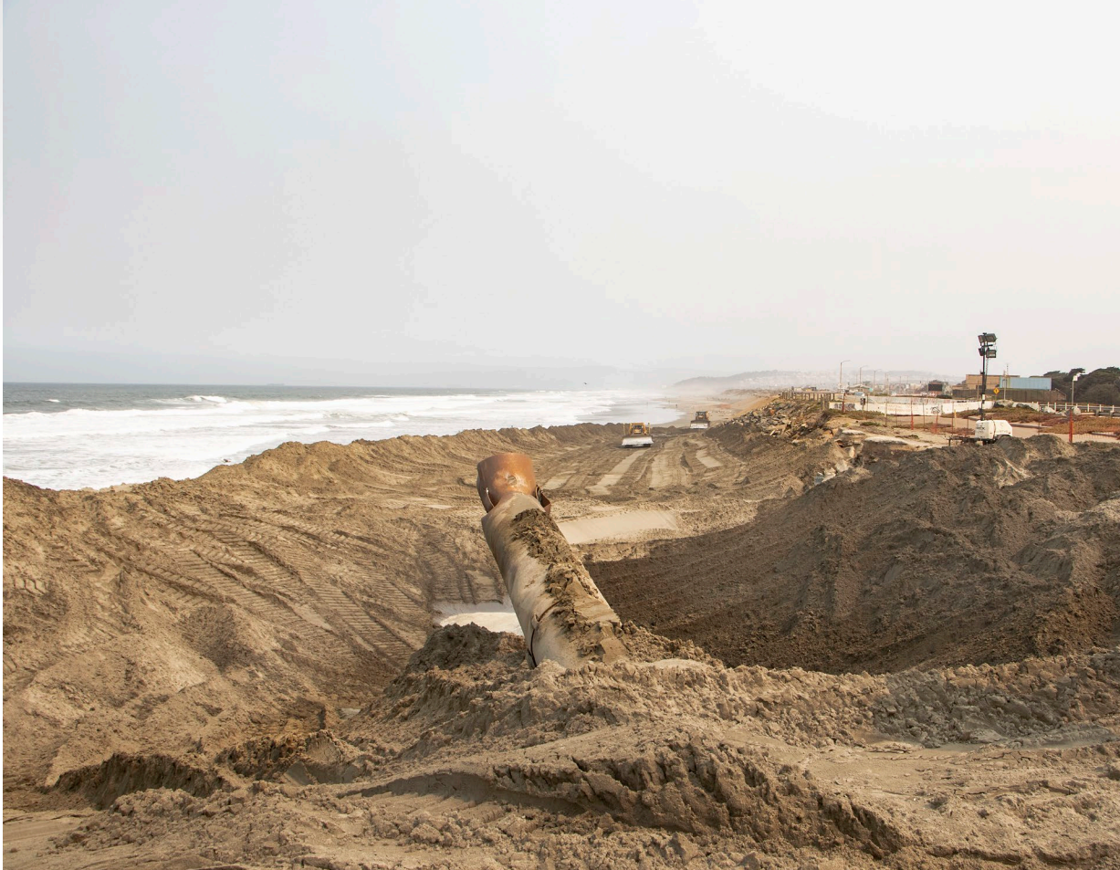
Photo of beneficial use project at Ocean Beach under construction.
