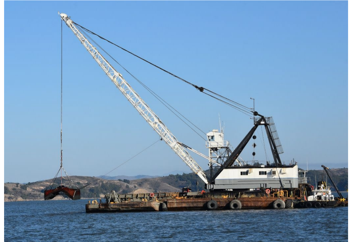
Photo of USACE maintenance dredging in San Francisco Bay with clamshell.
