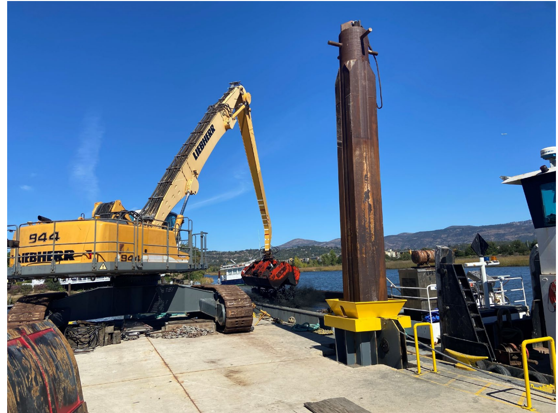
Photo of maintenance dredging of the Napa River from the Horton barge and dredge.
