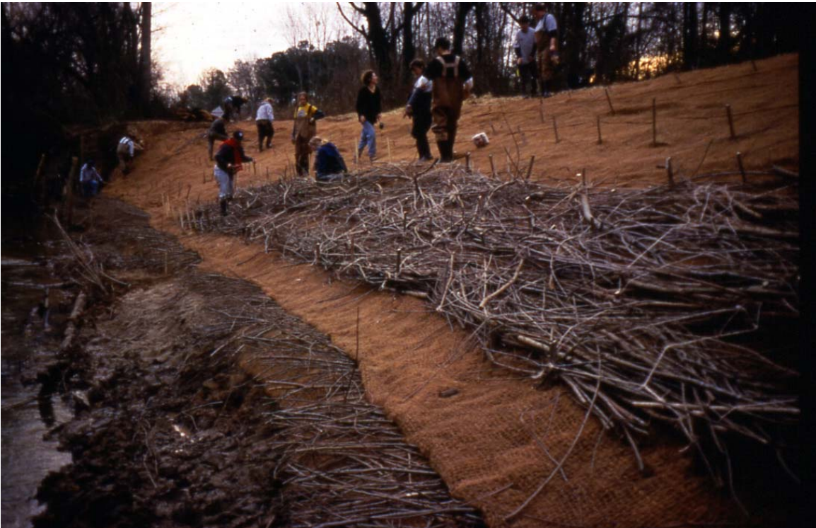
Figure 15C. Brush and Post Installation
