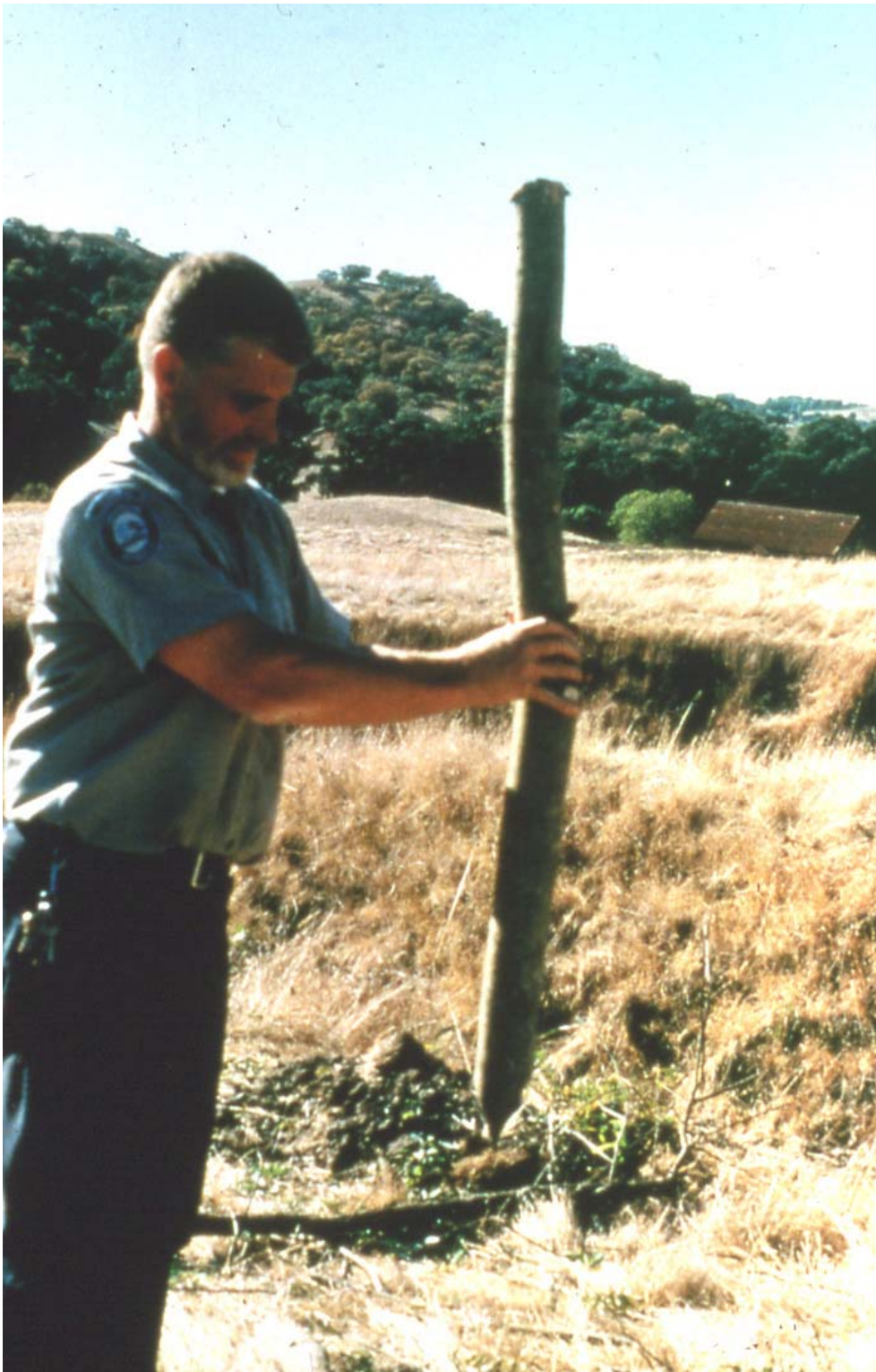
13 B Photo: Willow Post. Note planting end has been pointed for easy installation.
