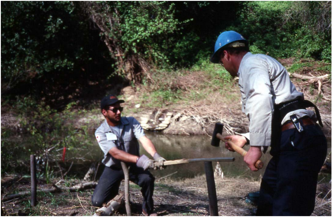
13 C Photo: Installing a willow or cottonwood post by hand.
