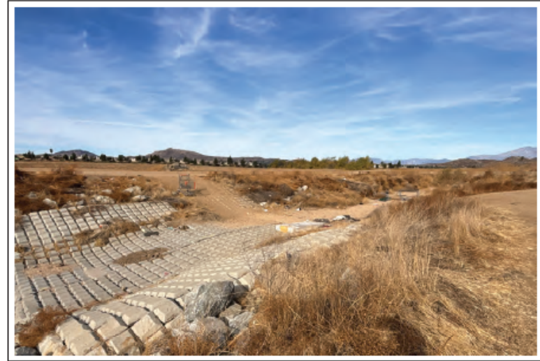
Photo 4. Upstream end of Drainage 1 facing northwest. December 19, 2024.
