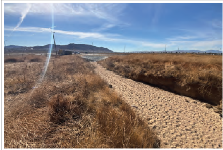
Photo 1. Downstream end of Drainage 1 facing the culvert under Cactus Avenue. December 19, 2024.
