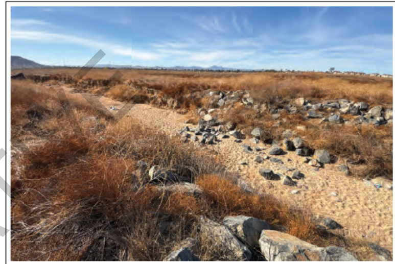
Photo 3. Middle of Drainage 1 facing southwest. December 19, 2024.
