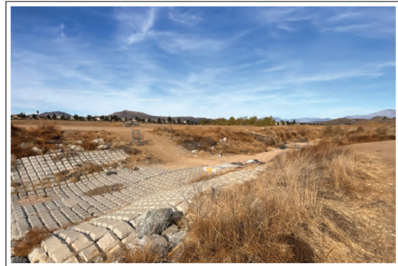
Photo 4. Upstream end of Drainage 1 facing northwest. December 19, 2024.
