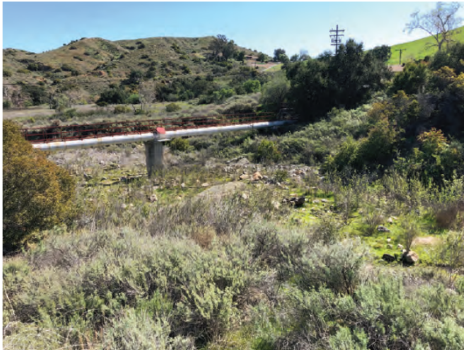
Figure 13: Santiago Creek at existing Irvine Lake pipeline
