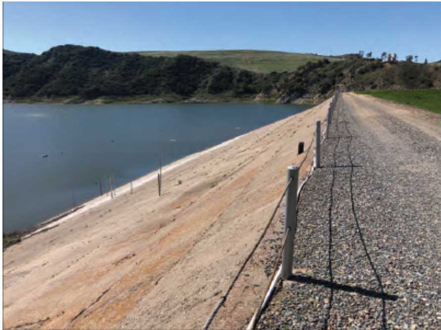
Figure 9 4: Santiago Creek Dam embankment
