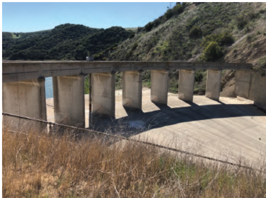
Figure 8: Existing Irvine Dam spillway structure
