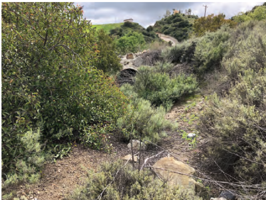
Figure 14: Pipe culvert leading into “Drainage 1”
