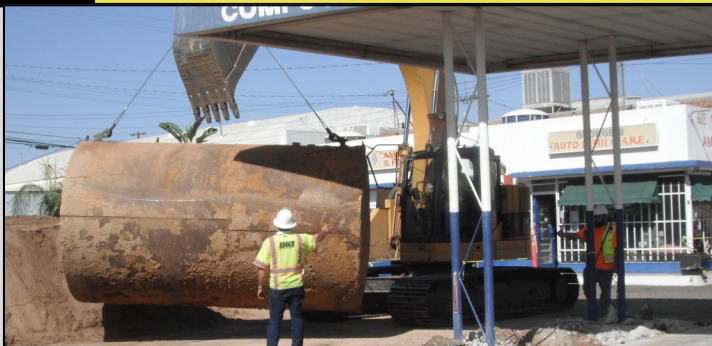
Photo: Removal of a UST at a former gas station
