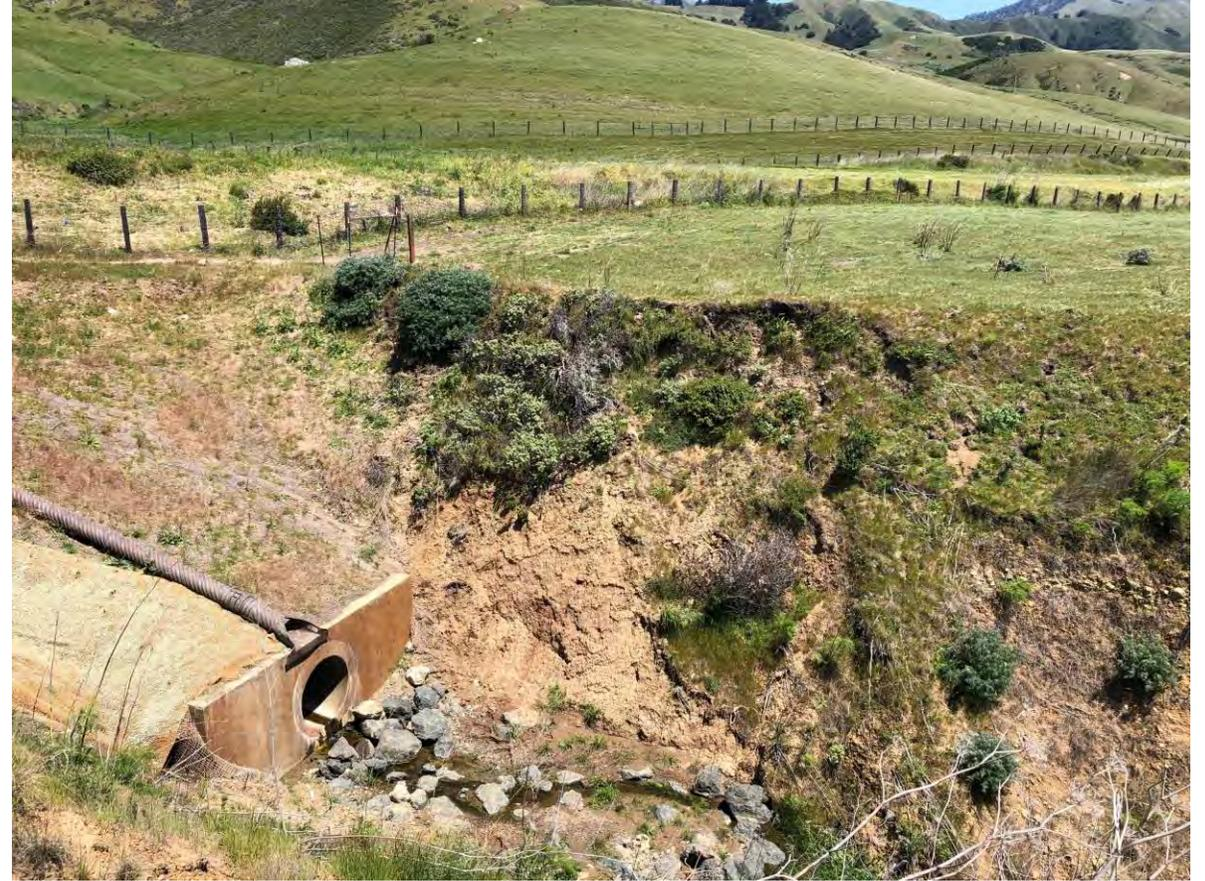
12 - Crossing of Existing Drainage with New Conveyance Pipeline (New pipeline will cross existing drainage along fence line, underground but above existing culvert.)
