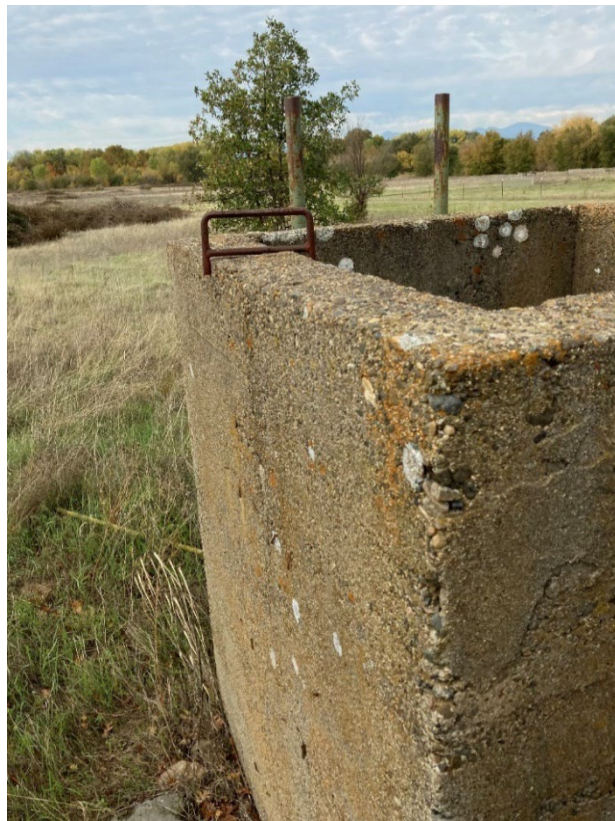
Irrigation box on former Tompkins Ranch, facing west toward Battle Creek.
