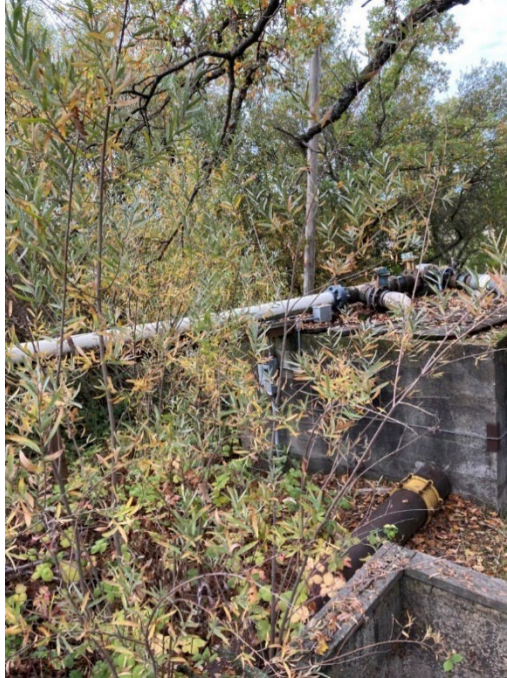
Diversion structure for stockpond on former Tompkins Ranch.
