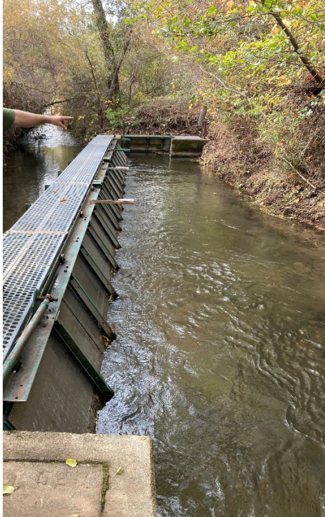
CDFW fish screen, with fish bypass pipe in background.
