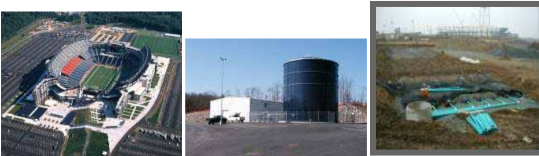
Figure 7.4. The reclaimed water facility in MA (center) serves a football stadium (left). The excess reclaimed water is periodically discharged in a vault to contribute to groundwater (right). The holding tank during peak seasons is shown in the center panel, right next to the treatment plant.
