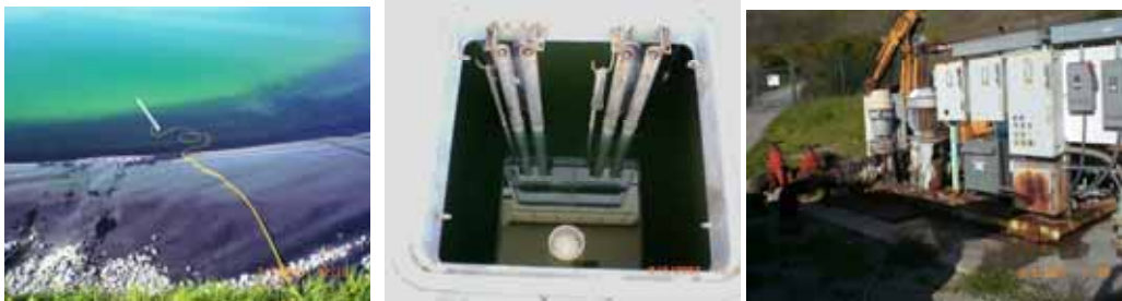
Figure 7.2. The CA plant site. The panel on the left shows the sampling tube submerged in the storage reservoir (pool), the center panel shows the chlorine contact basin, and the panel on the right shows the pumping station for moving water up to the storage reservoir and out to the distribution system.
