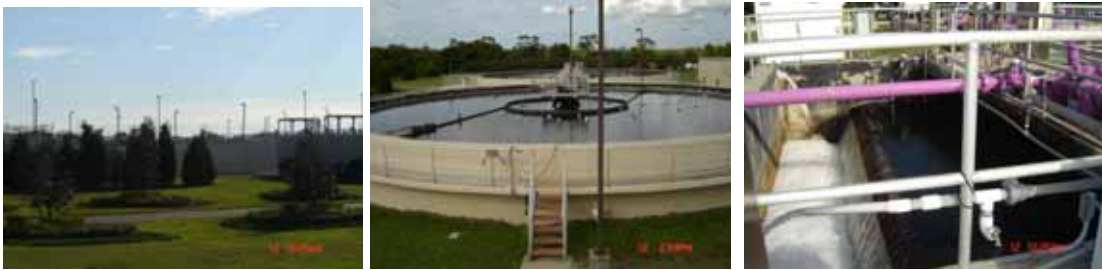
Figure 7.3. The FL plant. The panel on the left shows the plant from the outer perimeter of the grounds, the center panel shows the clarifier, and the panel on the right shows finished and postchlorinated water. The plant has a total of six clarifiers.
