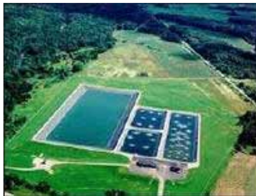
Figure 3.5. Lagoons for wastewater treatment.
