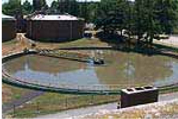
Figure 3.2. Primary settlement tank.
