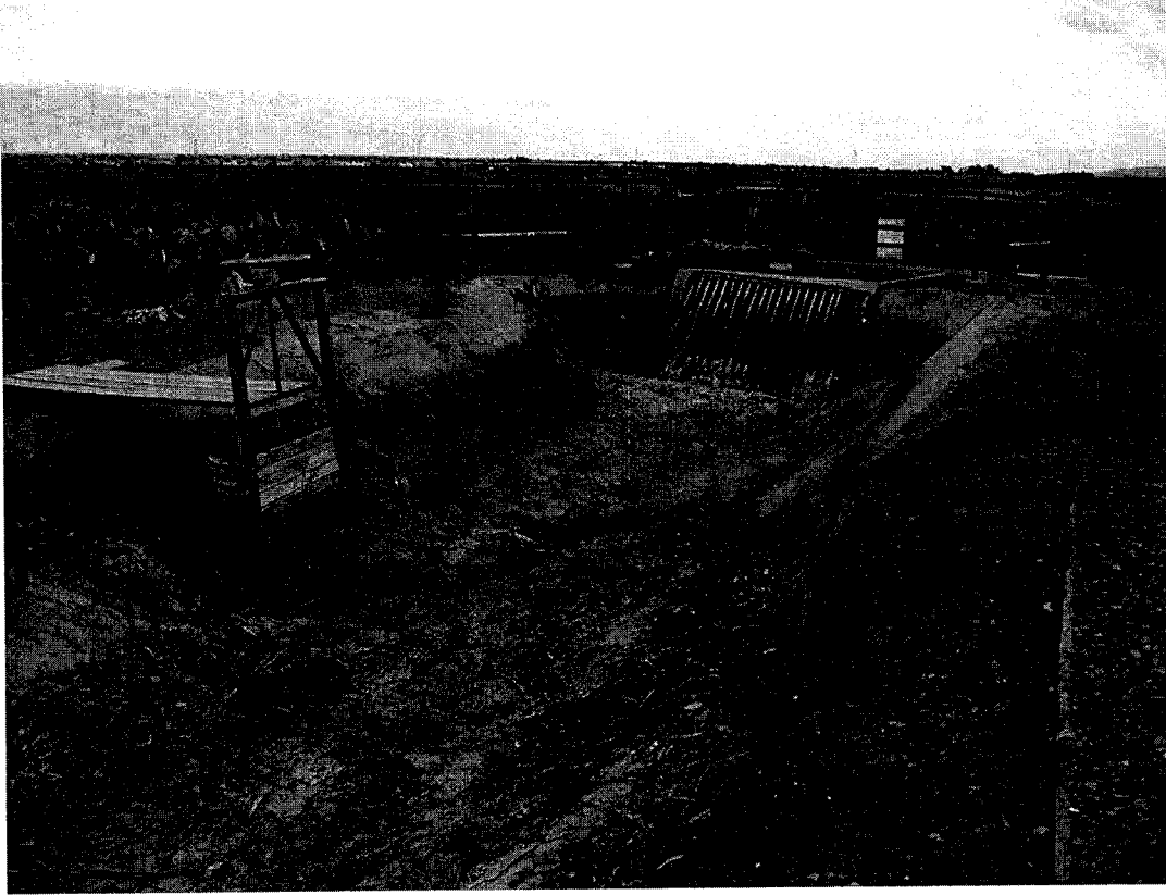
FIGURE 4-1 120 Spillway Visual Monitoring Location
