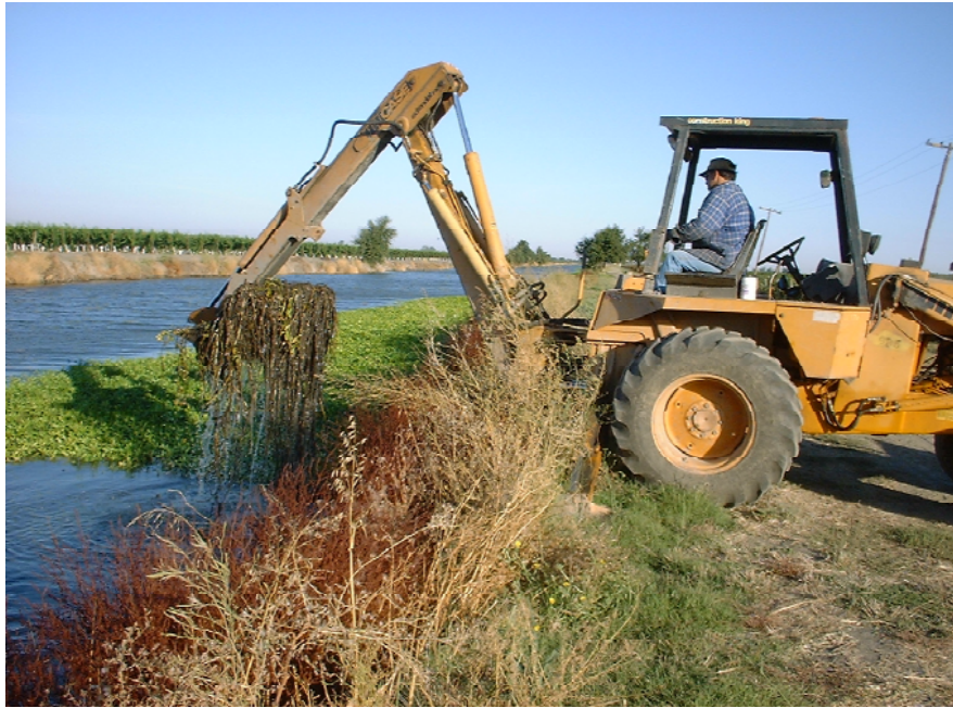
Figure 4.1. Mechanical removal of floating weeds at RD999.
