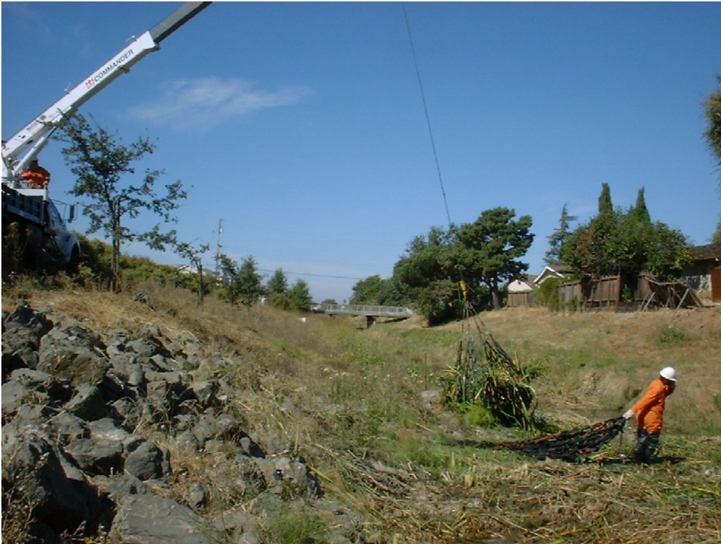
Figure 4.7. Hauling tules out of the removal site using a crane.
