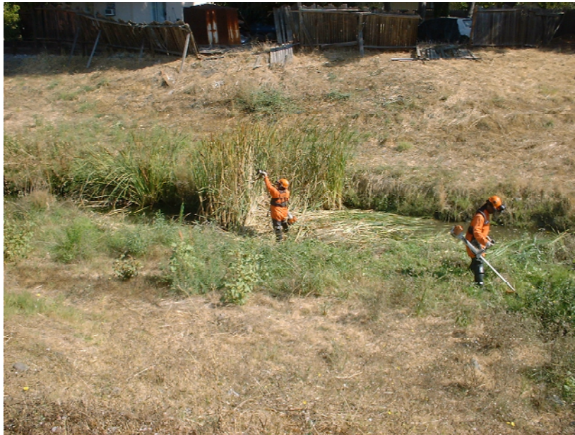
Figure 4.6. Manual removal of tules using power brush cutters.
