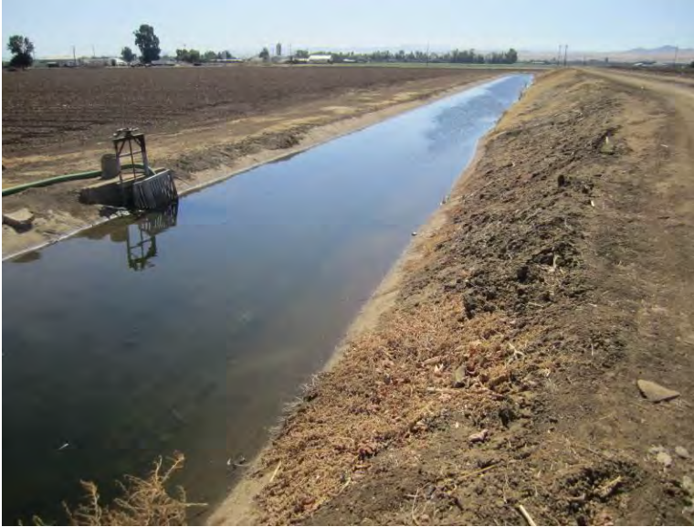
Photo 1. Northernmost reach of 45 Canal within BBID, looking southwest.
