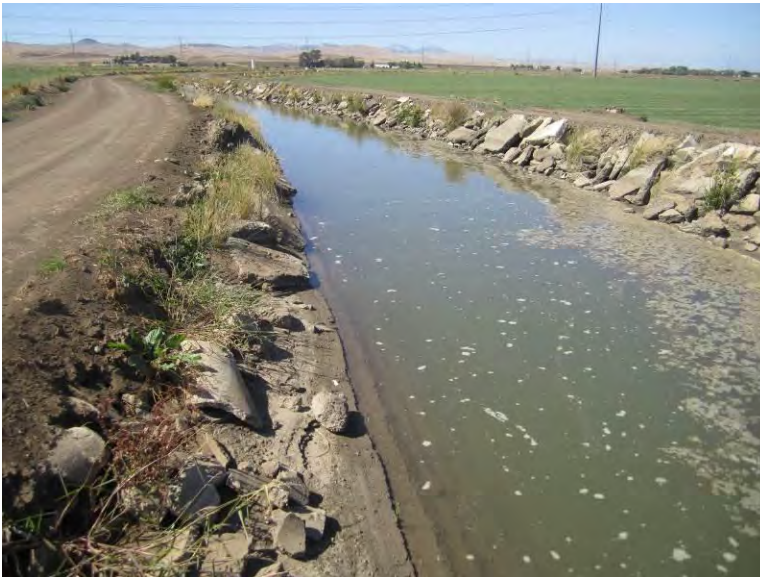
Photo 2. 120 Canal east of Mountain House Road within BBID, looking northwest.
