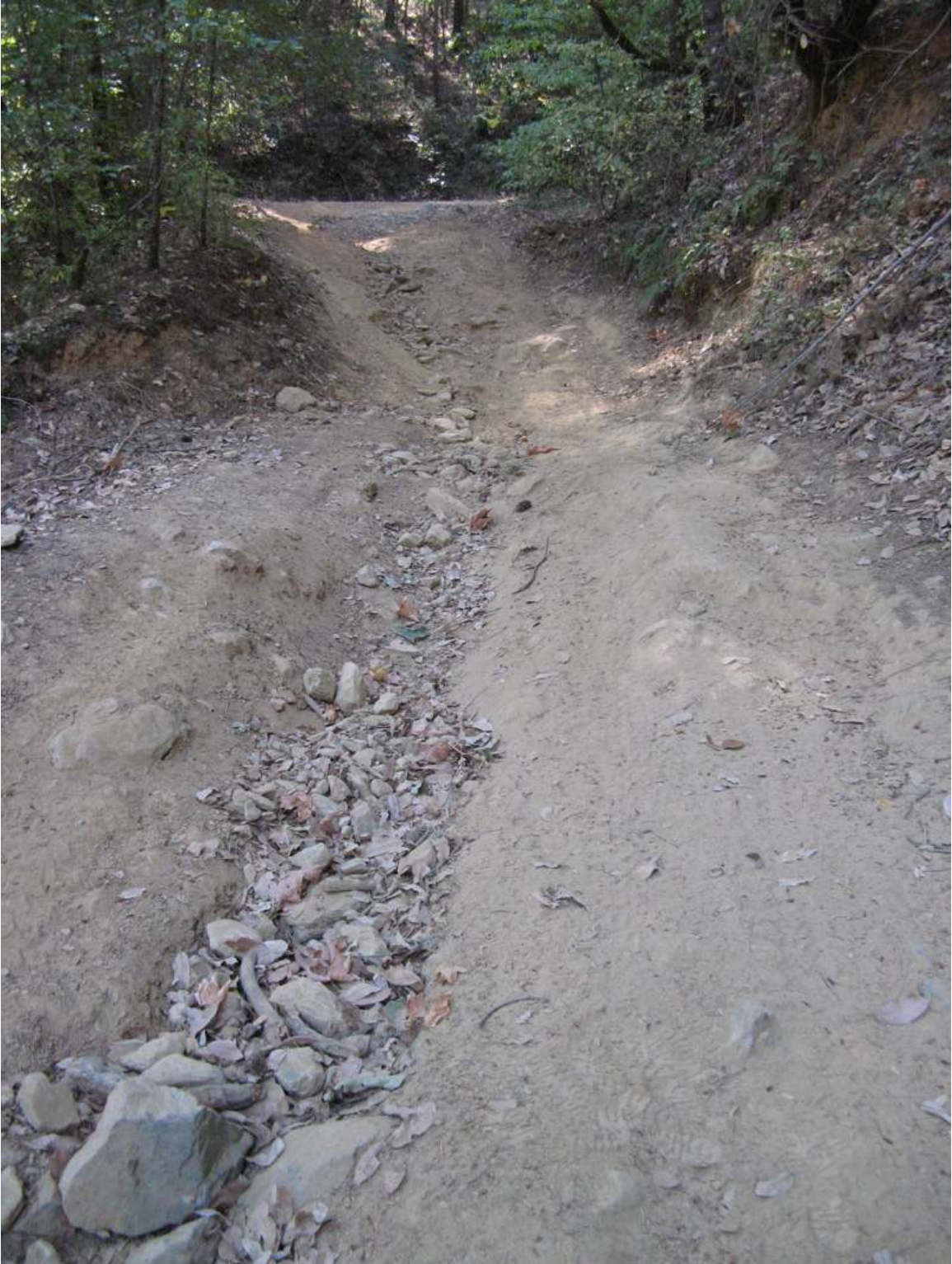
OHV approach to Rock Creek. This trail funnels sediment several hundred feet with no effort to keep the sediment out of the creek. This is a designated OHV trail.
