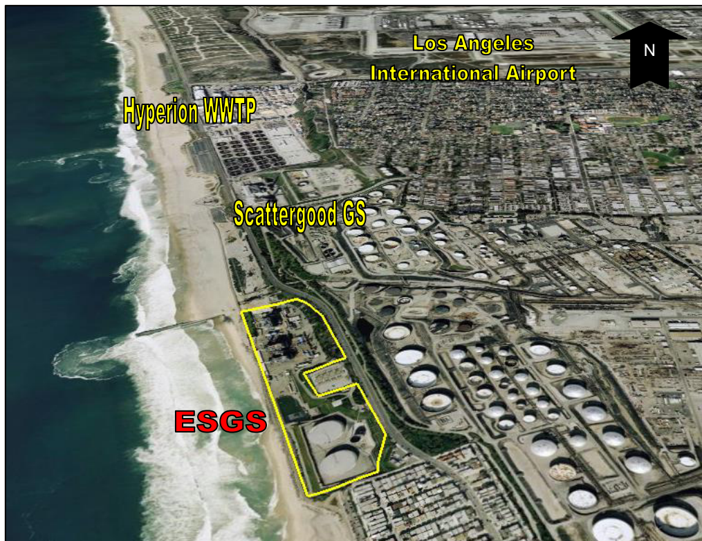
Figure D-1. General Vicinity of El Segundo Generating Station
