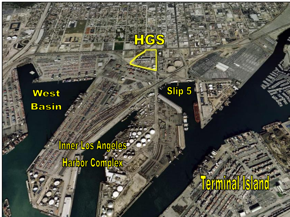
Figure E-1. General Vicinity of Harbor Generating Station
