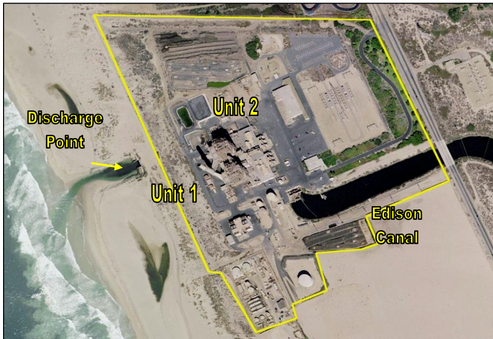
Figure H-2. Site View
