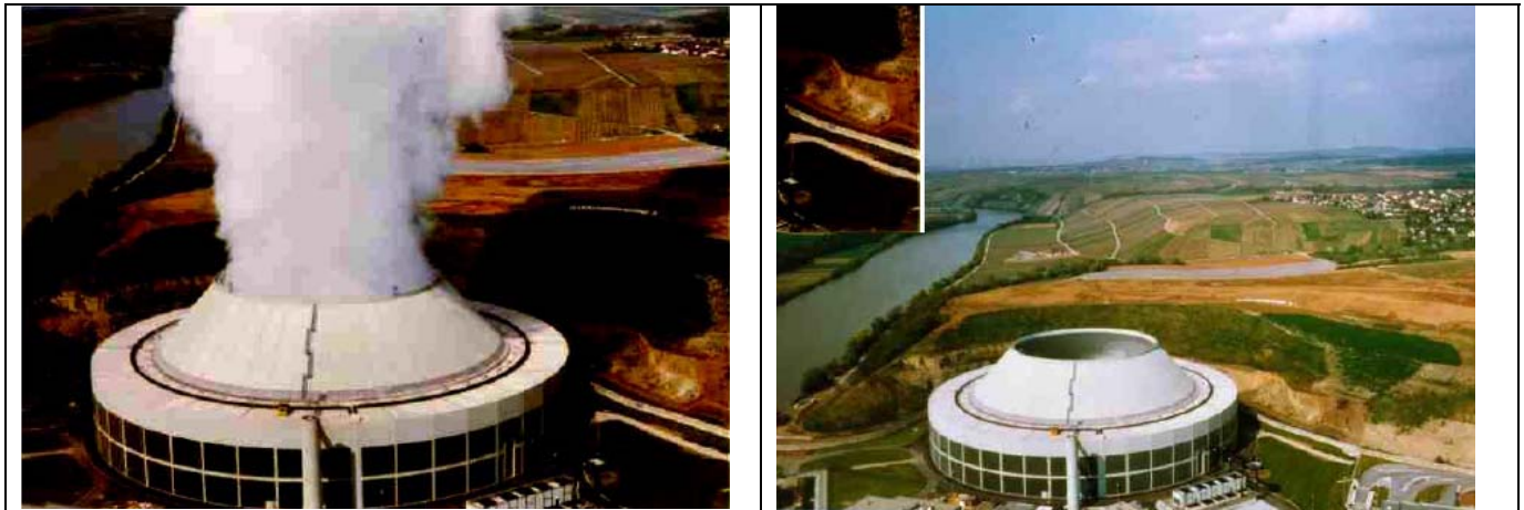
500 ft. diameter, 160 ft. tall plume-abated round wet tower, GKN2 1,300 MW nuclear reactor (Germany), 1 billion gal/day cooling water flow. Left photo – plume abatement off. Right photo – plume abatement on. Source: BALCKE GmbH
