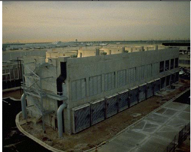
Operational plume-abated tower, ~50 ft. tall – Chicago O'Hare Airport Source: P. Lindahl – Marley presentation, May 2002.
