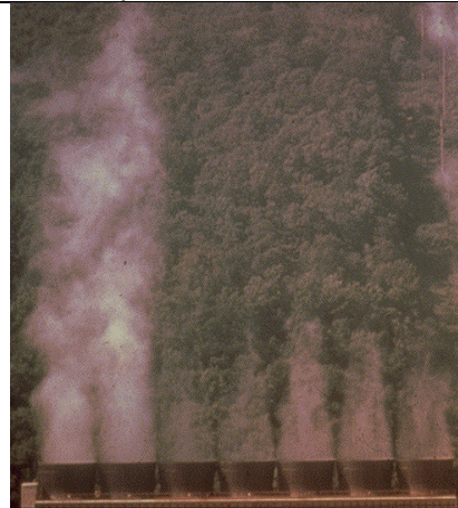
Effect of plume abatement function – Plume abatement off, left two cells. Plume abatement 100% on, adjacent two cells. Source: P. Lindahl – Marley presentation, May 2002.
