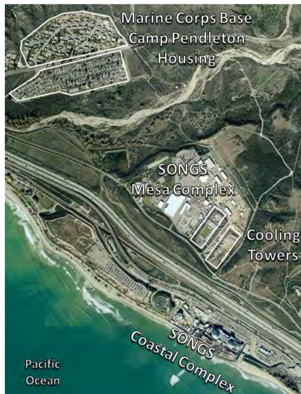
Figure 3.6 Location of MCBCP Housing near Cooling Towers
