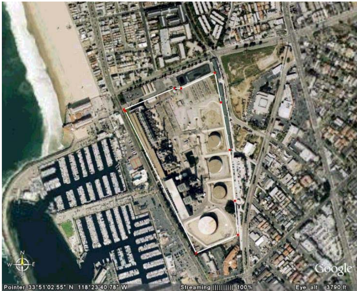
Figure B-99 Redondo Beach Power Station: Boundary and Neighborhood
