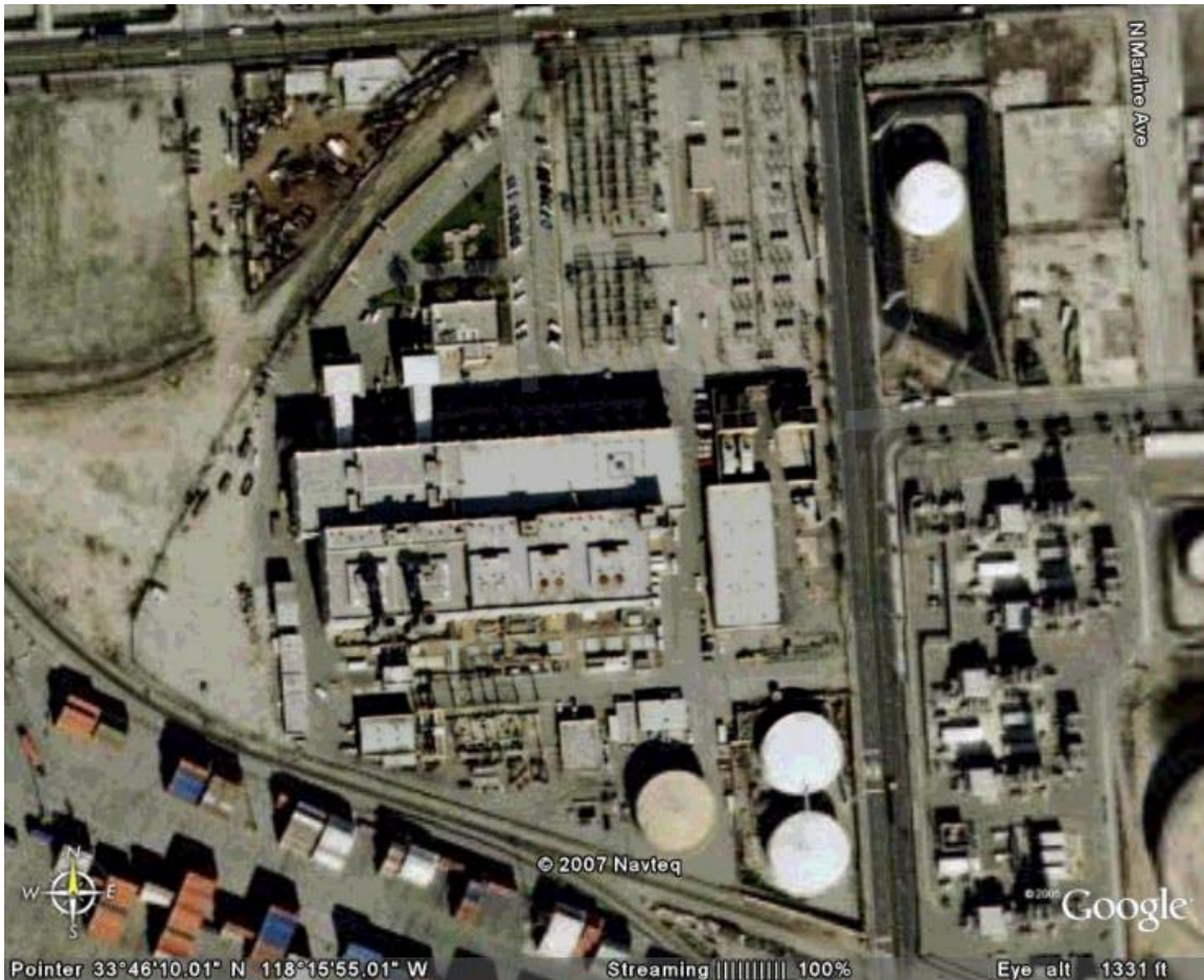
Figure B-54 Harbor Generating Station Site View
