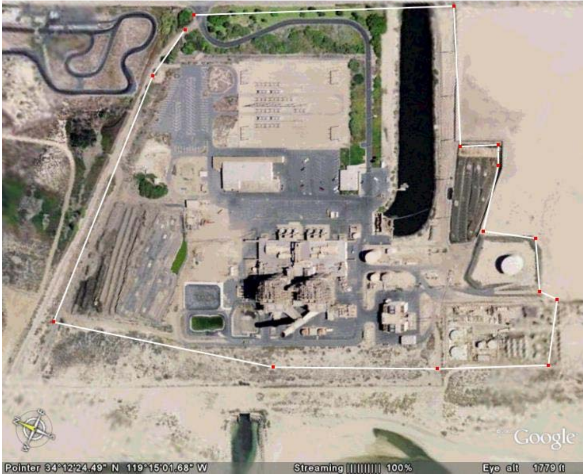
Figure B-62 Mandalay Power Station Site View
