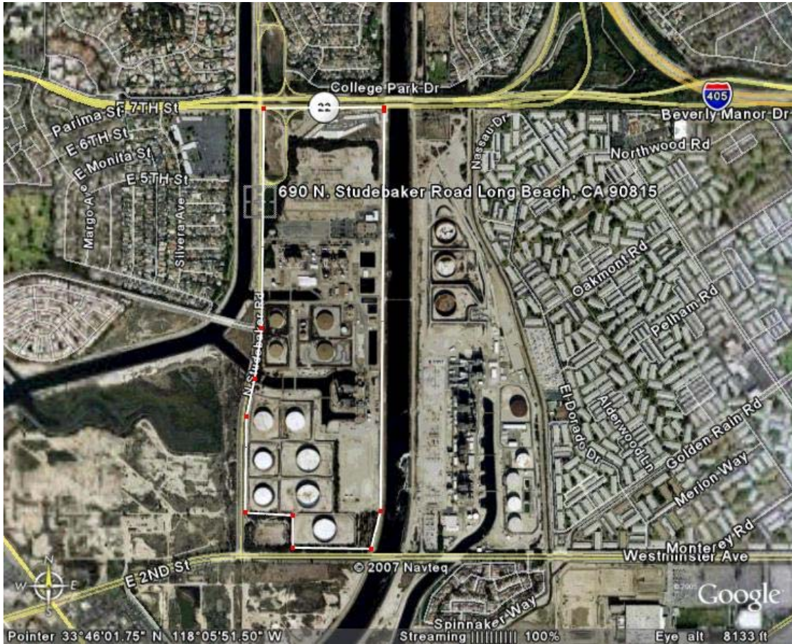
Figure B-1 Alamitos Generating Station—Boundaries and Neighborhood
