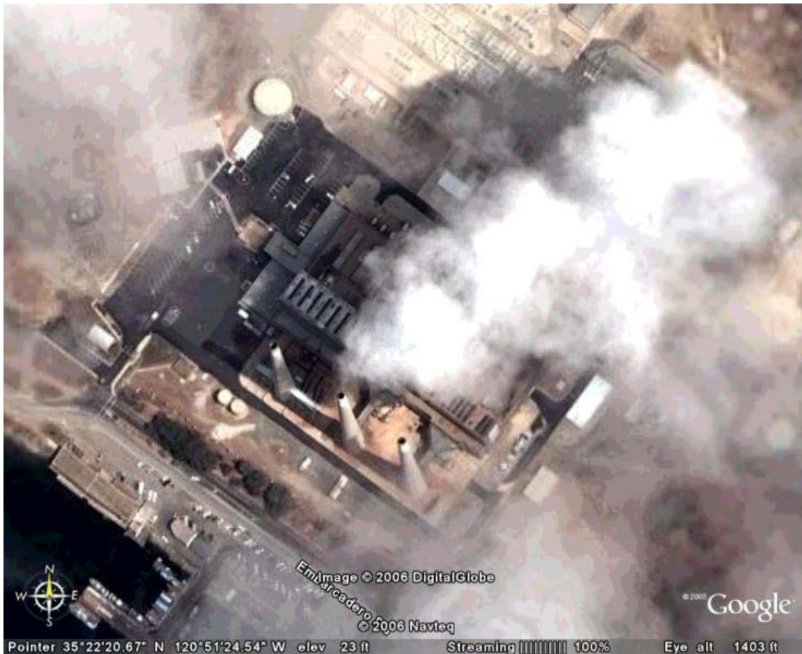
Figure B-68 Morro Bay Steam Plant Site View
