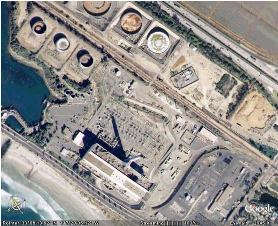
Figure B-26 Encina Site View
