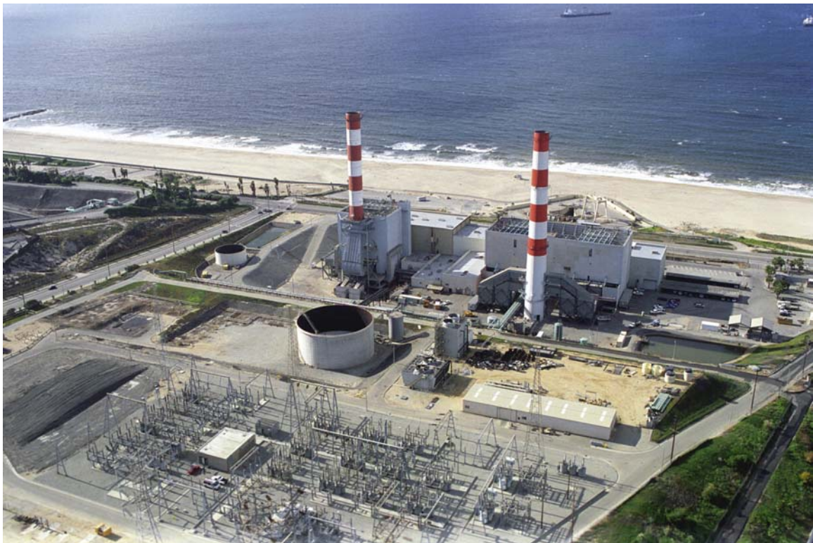
Figure B-115 Scattergood Generating Station: Site View
