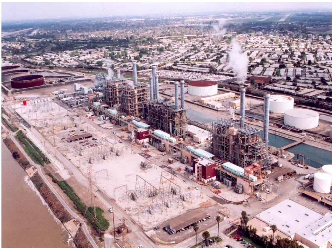
Figure B-37 Haynes Generating Station: Site View
