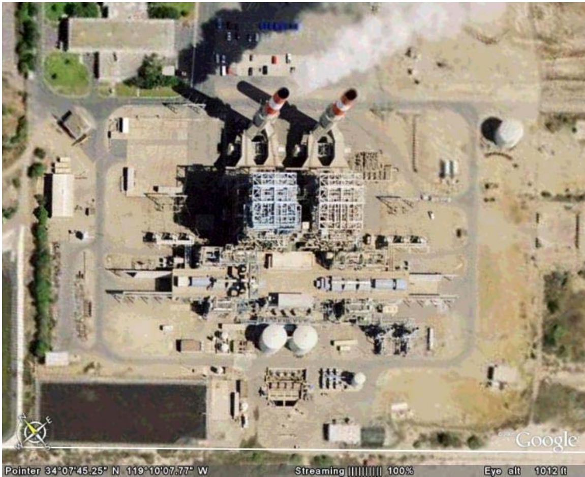
Figure B-81 Ormond Beach Power Station: Site View
