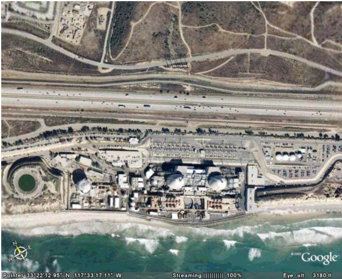
Figure B-104 San Onofre Nuclear Power Station Site View
