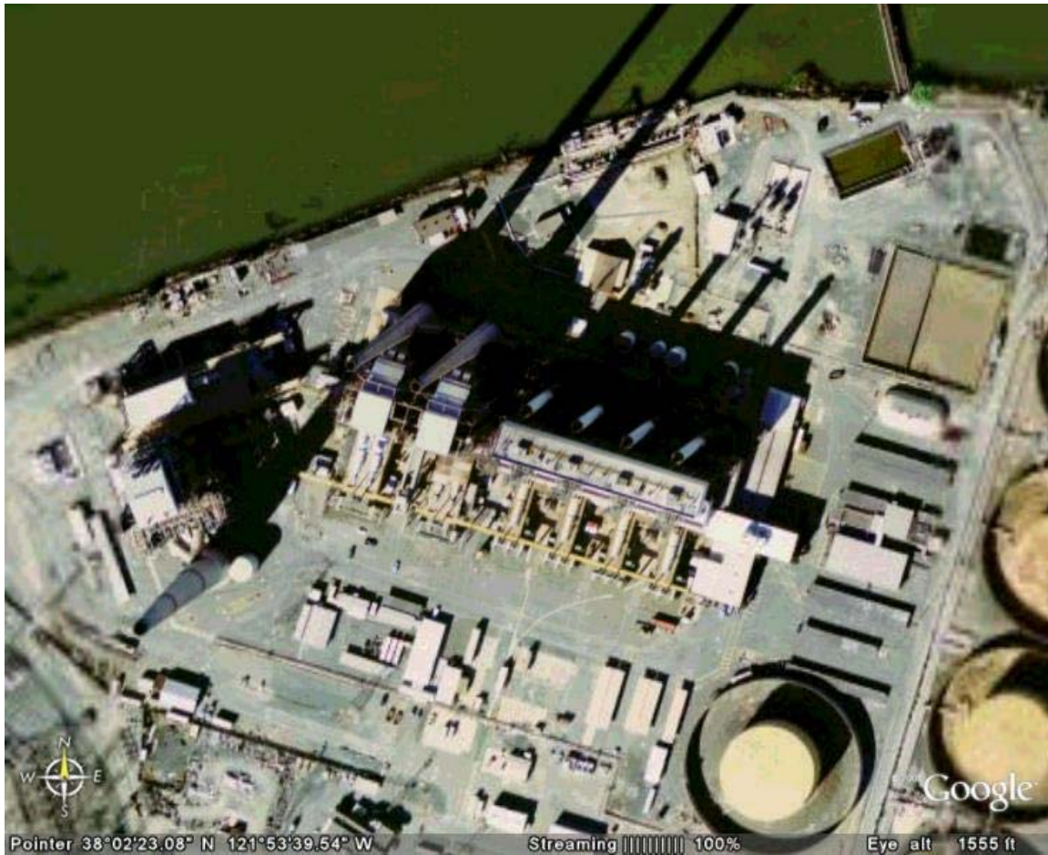
Figure B-87 Pittsburg Generating Station: Site View
