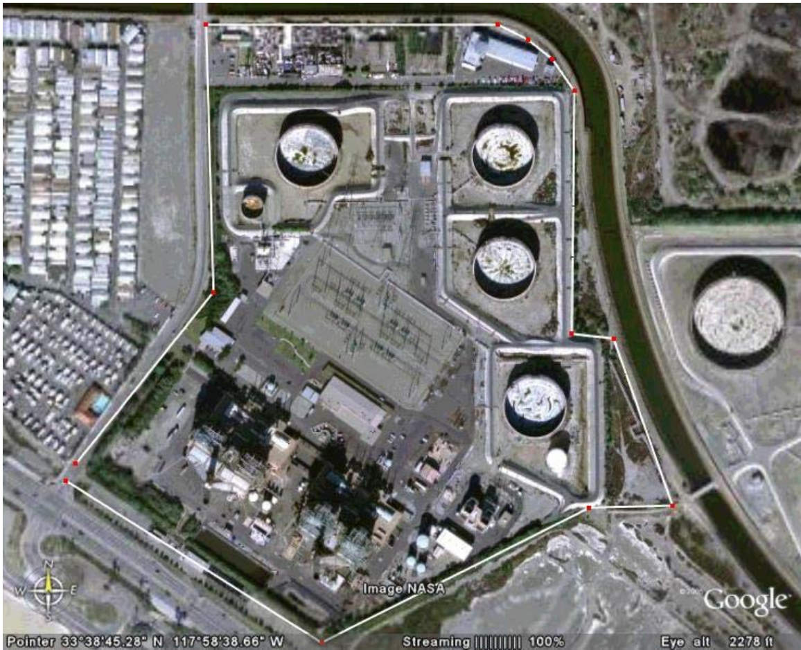
Figure B-48 Huntington Beach Generating Station: Site View
