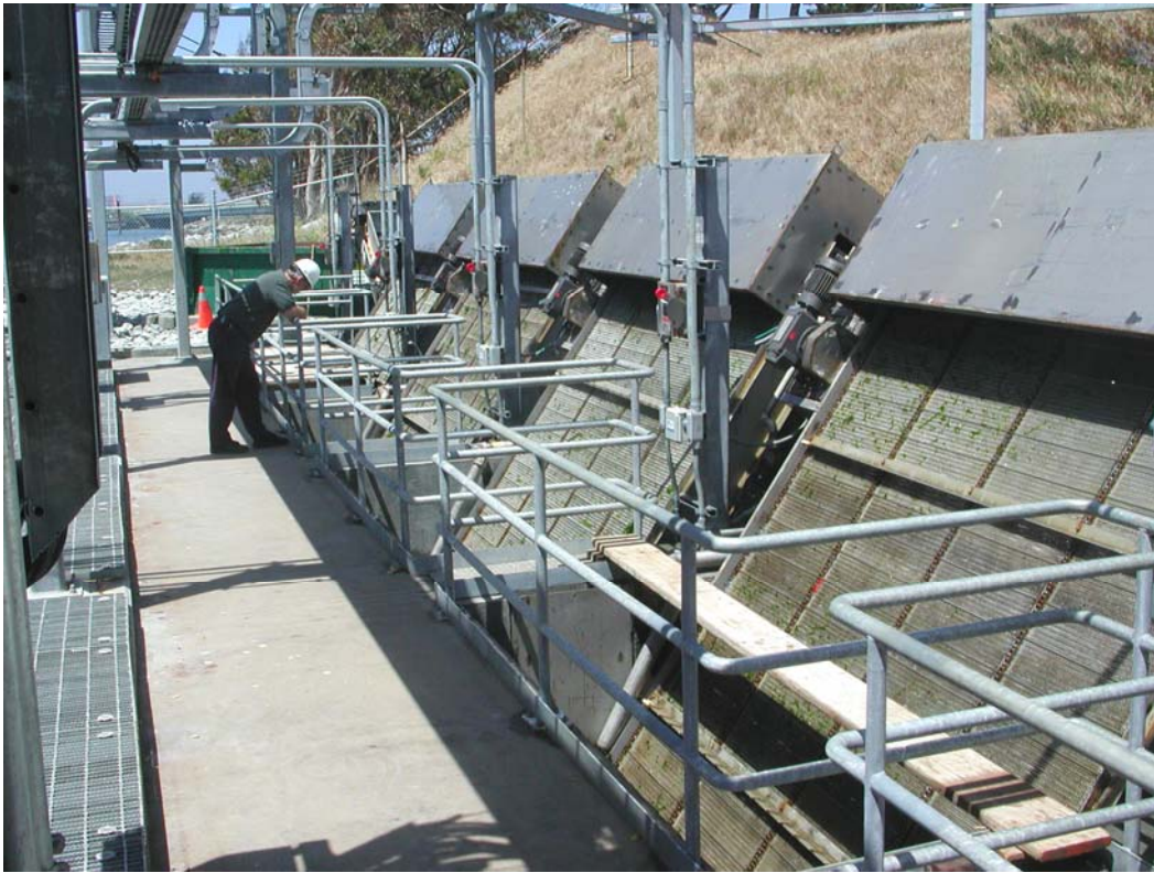
Figure 2-5. Units 1&2 traveling screens. Four of the six screens are shown.
