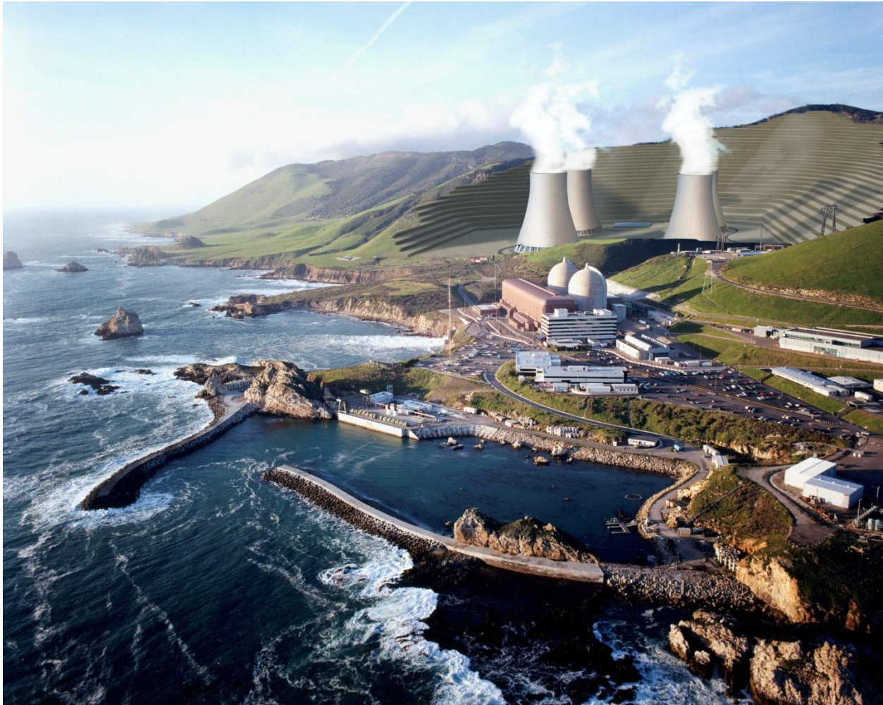
Figure 4.3-16. Wet Natural Draft Cooling Site Configuration
