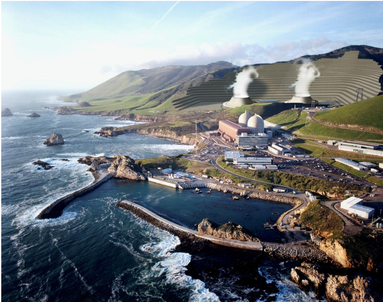
Figure 4.3-20. Wet Mechanical (Forced) Draft Cooling Site Configuration
