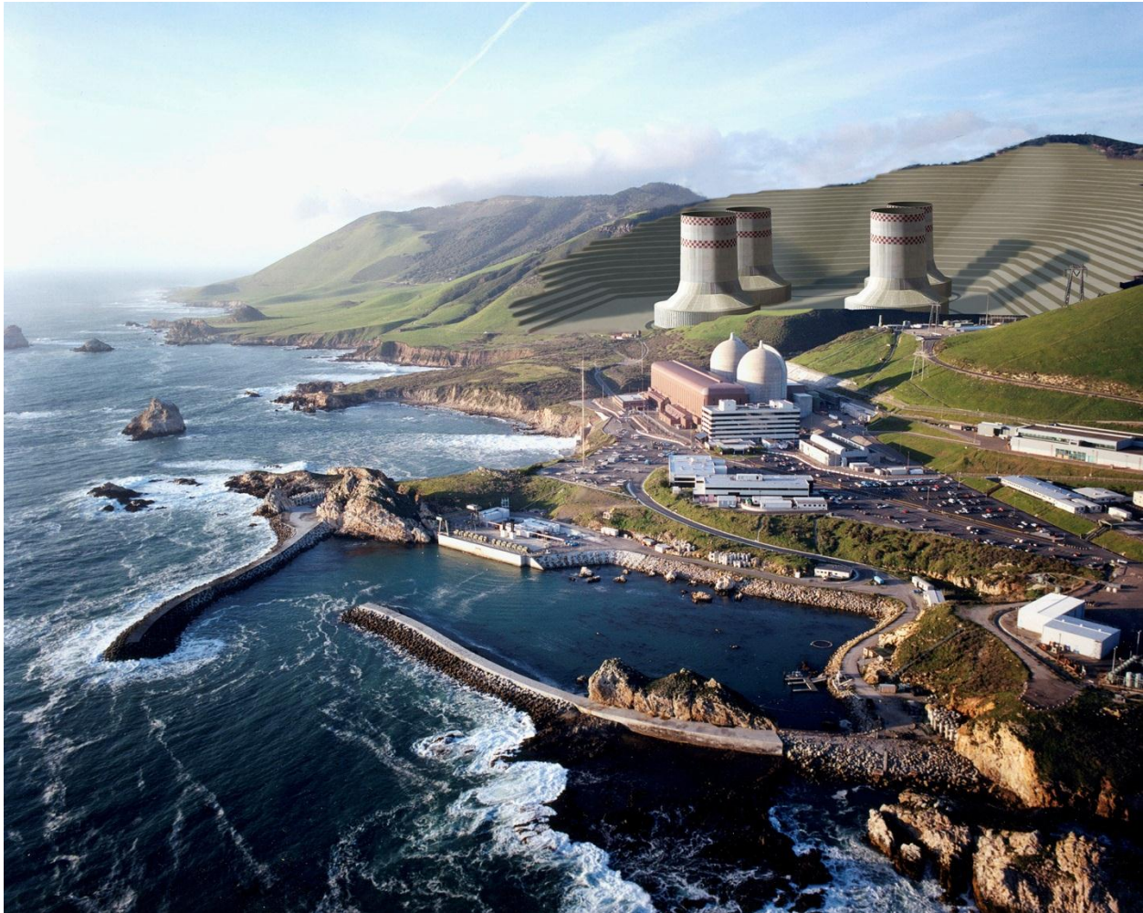
Figure 4.3-9. Passive Draft Dry/Air-Cooling Site Configuration
