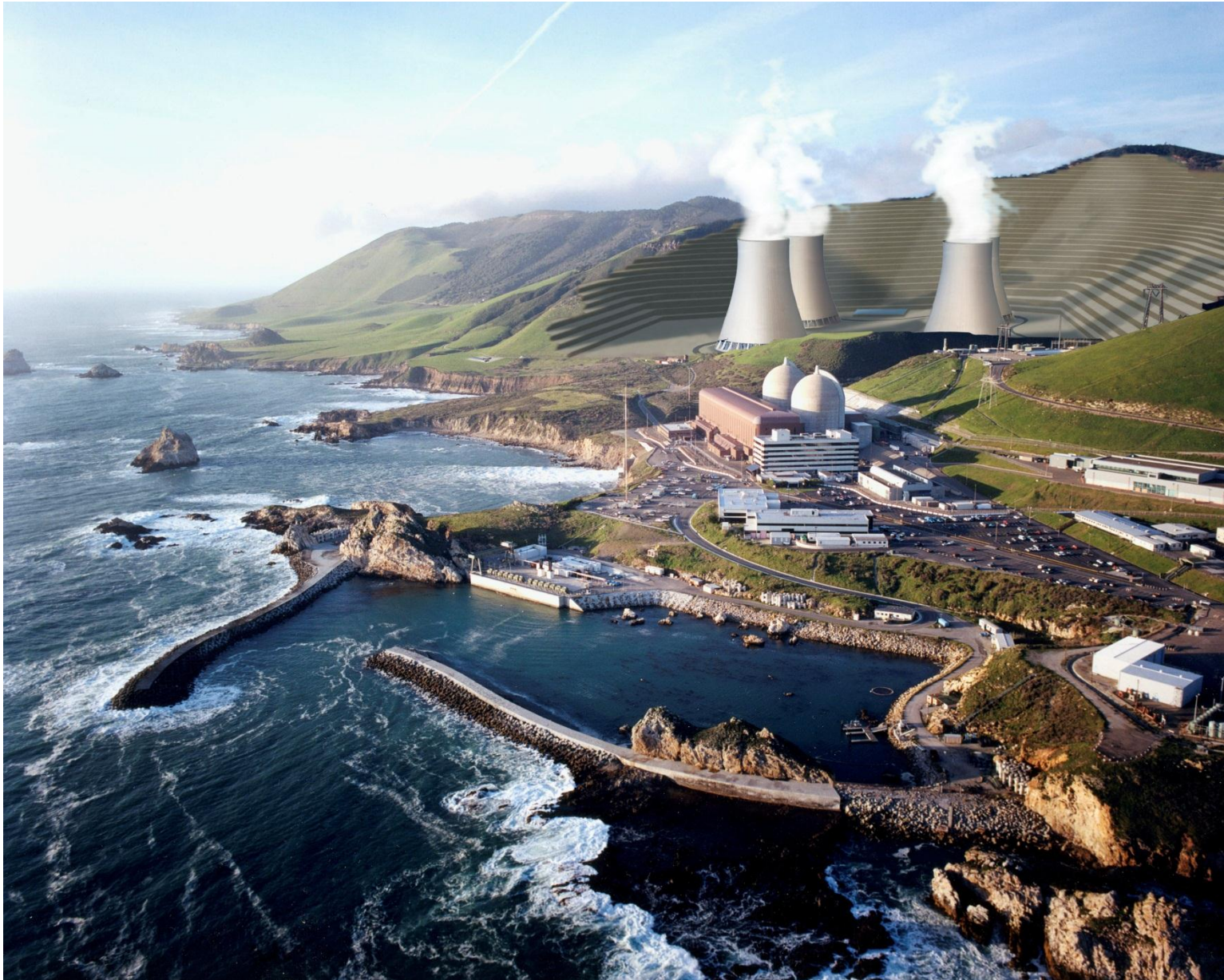
Figure 4.3-4. Plant Site Rendering Showing Wet Natural Draft Technology
