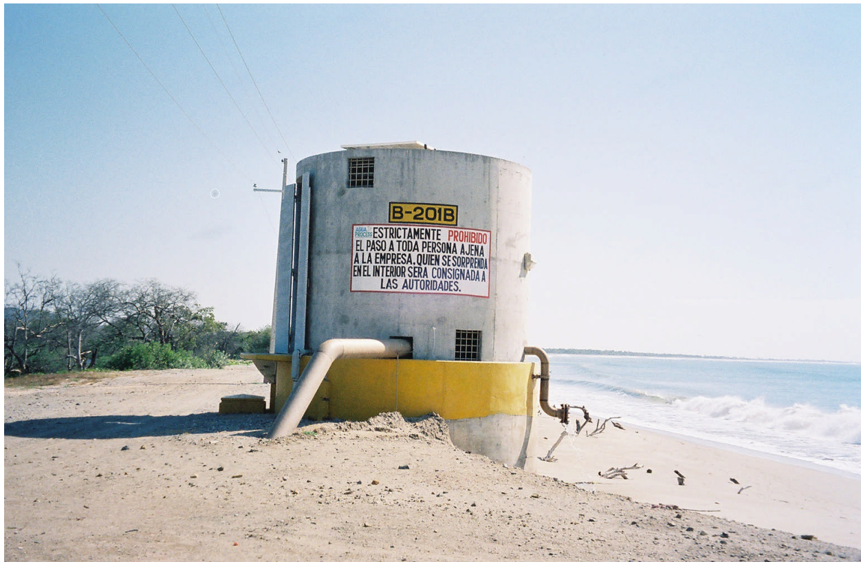
Figure 2 – 3.8 MGD Horizontal Seawater Intake Beach Well
