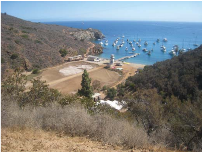
5-2c. Retention Basin- Cherry Cove
