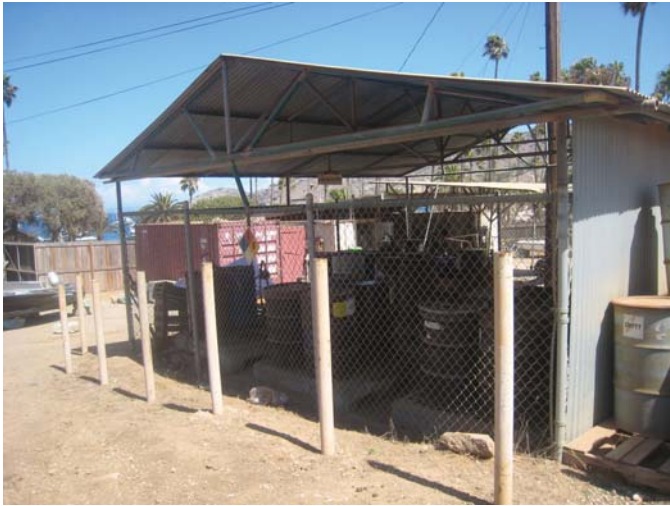
5-2a. Covered Hazardous Materials Area- Two Harbors
