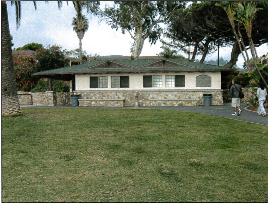
Photo - Rebuilt restroom facility.
