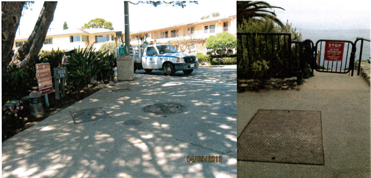
Photo - Jasmine Street Diversion Unit/Lid to sump pump.
