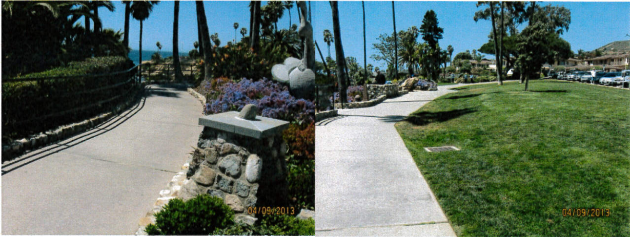
Photos - Pathways and surrounding terrain are tilted toward a depressed bioswale for infiltration.
