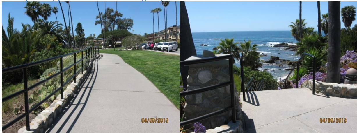
Photos – Curbs, railings and improved stairs to beach ensure visitors are not destroying the bluff tops. Tilted pathway push sheet flows to the grassy area for infiltration.
