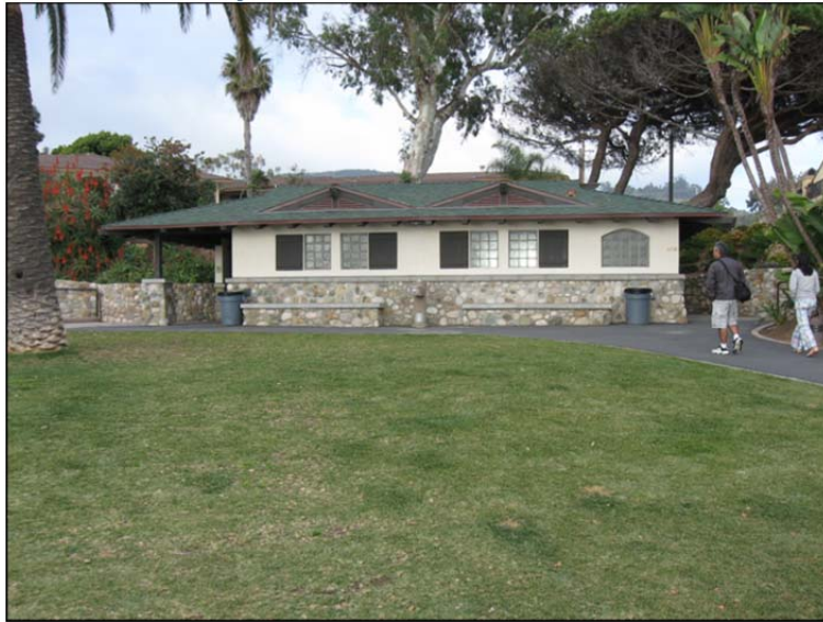
Photo – Rebuilt restroom facility.
