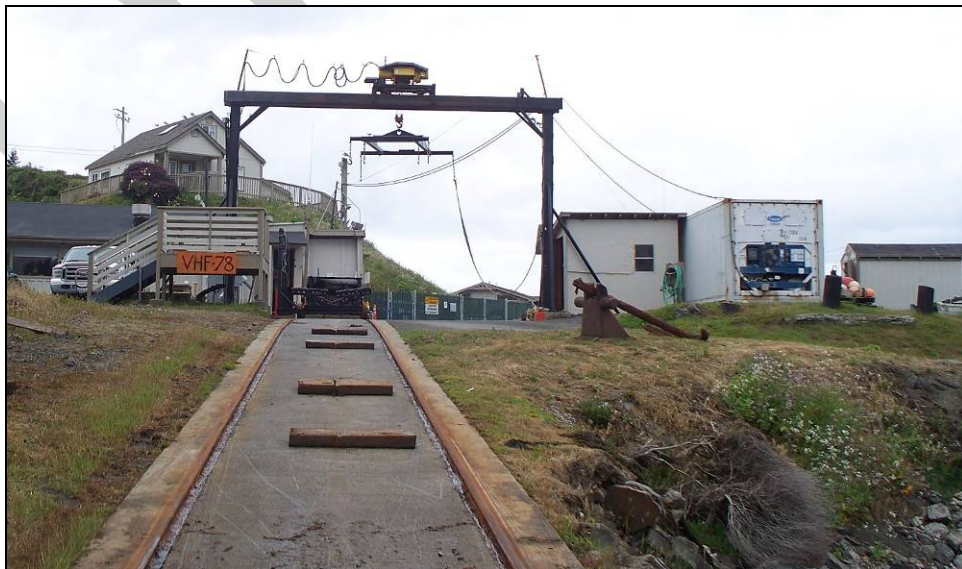
Photo 4. Boat Launch Rails, northwestern view.
