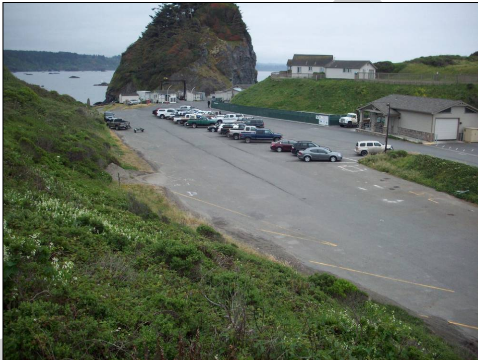
Photo 1. Southeastern view of the main parking lot, from Lighthouse Road.
