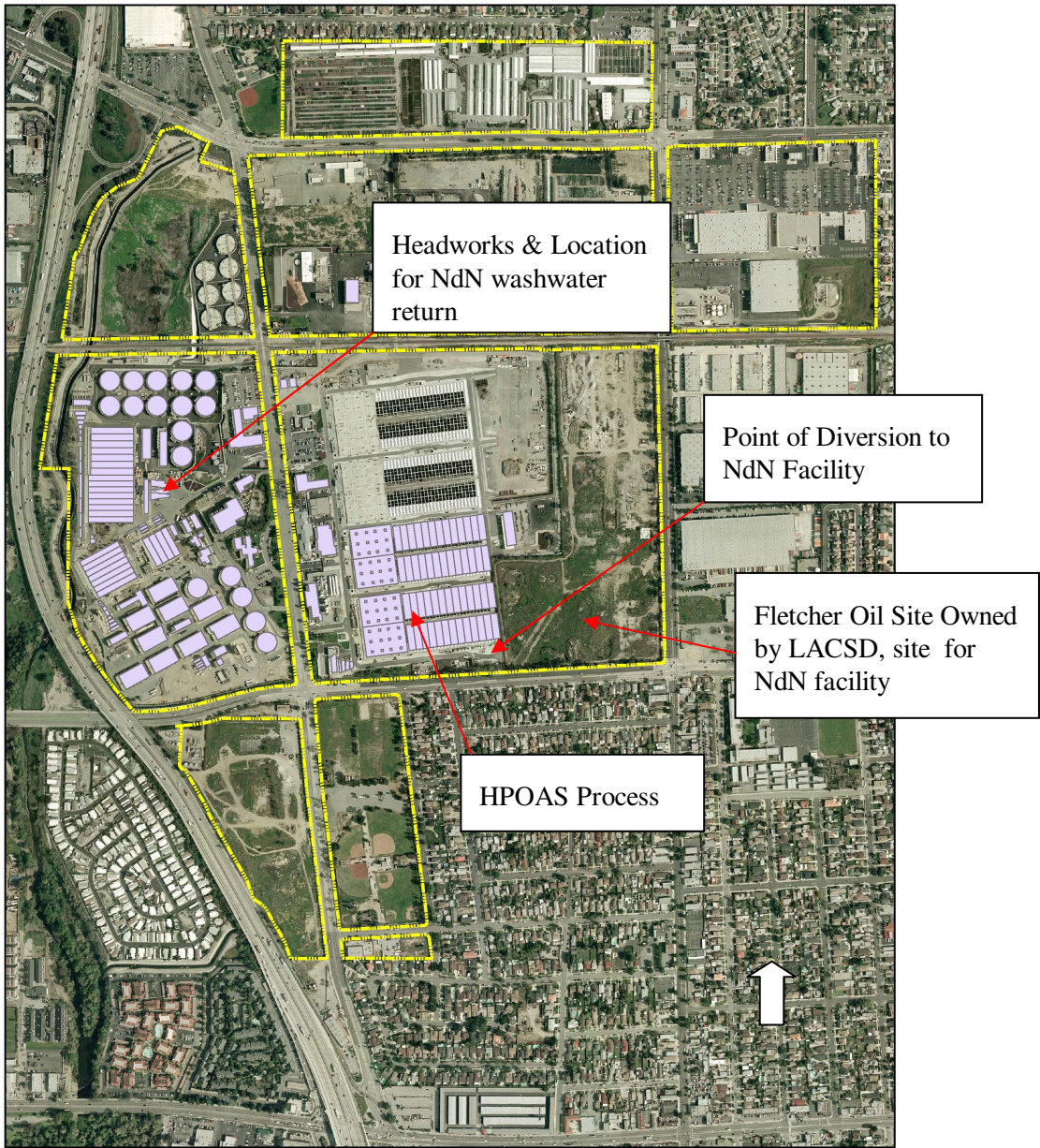
Figure 3-1 Aerial View of JWPCP
