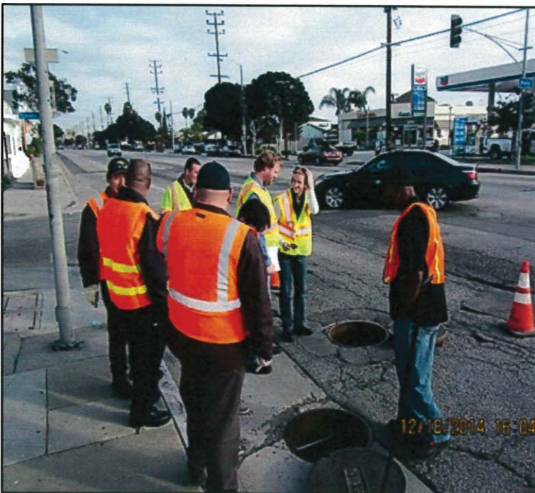
Photo 31: Sewer siphon inspection site (view 1)
