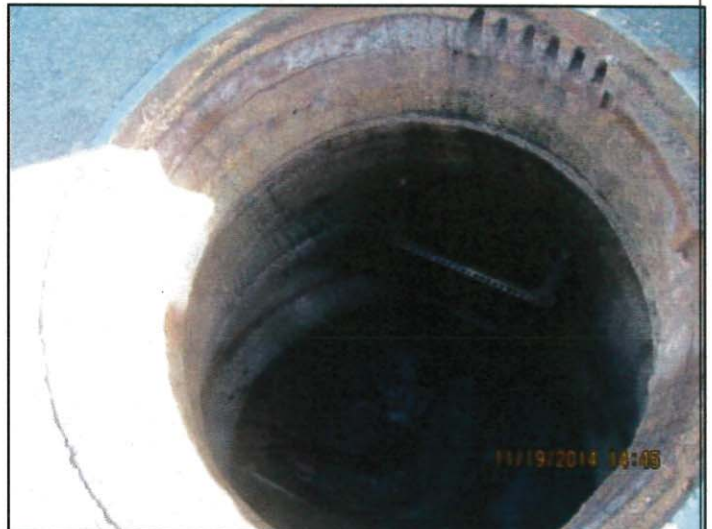
Photo 18: Former root blockage SSO site manhole (view 2)
