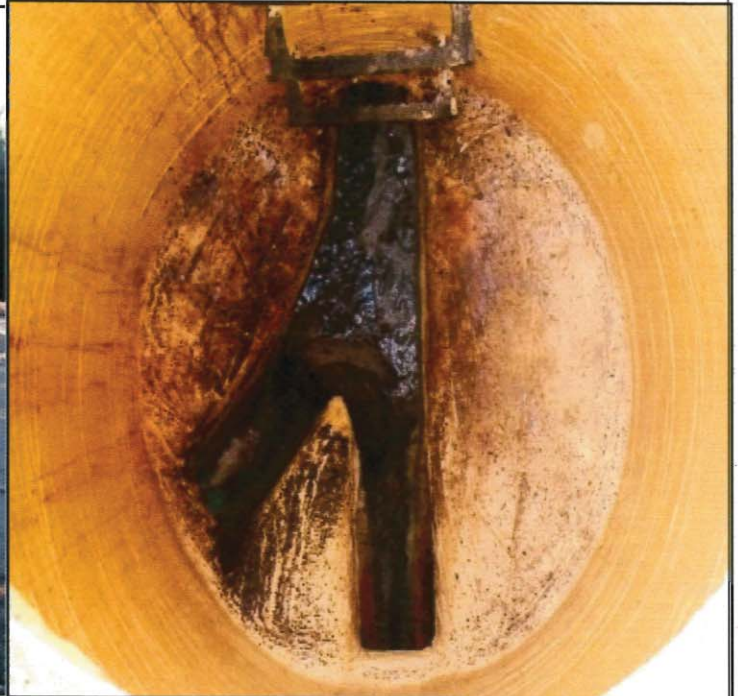
Photo 22: View of manhole, pipeline and rag
