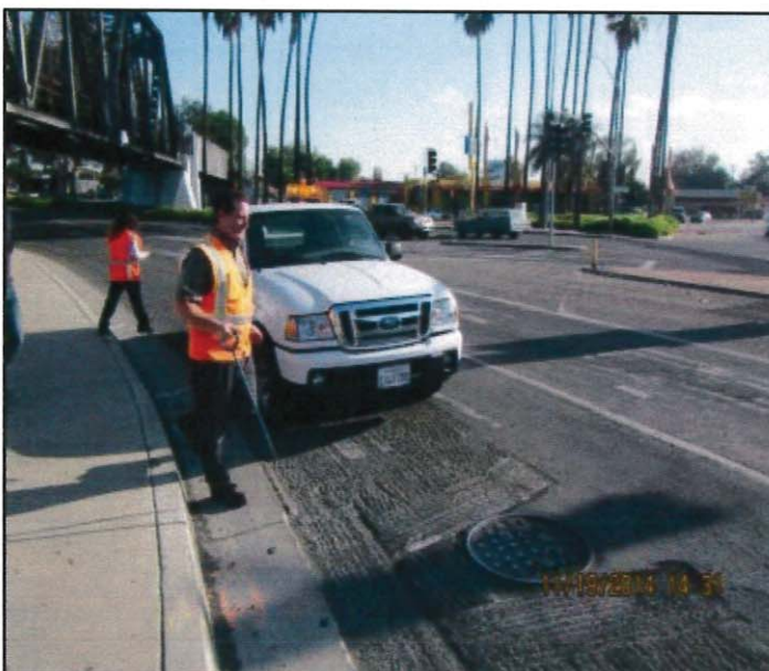
Photo 11: Miller opening manhole for capacity inspection
