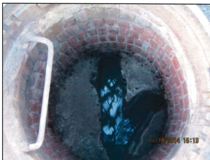
Photo 26: View of mainline sewer in this location (view 2)
