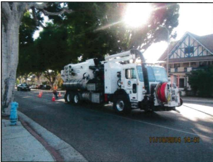
Photo 15: Former root blockage SSO site (view 1)
