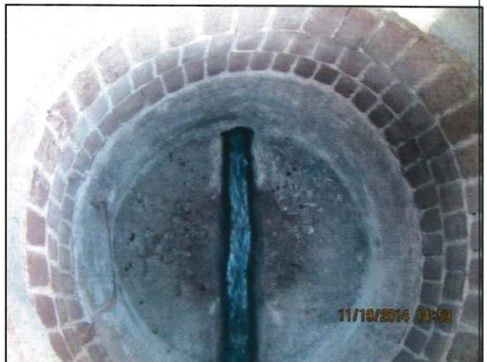
Photo 20: View of manhole in this location
