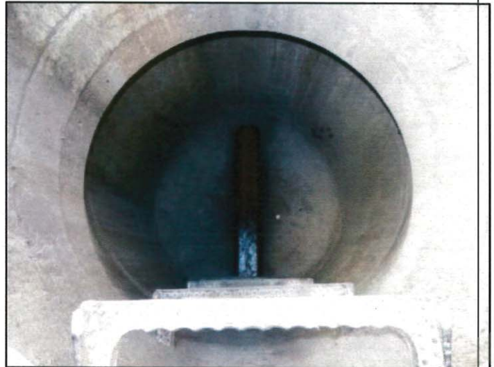
Photo 10: FOG sewer line inspection (view 2)
