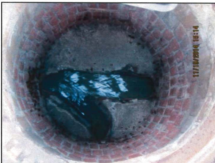
Photo 25: View of mainline sewer in this location (view 1)
