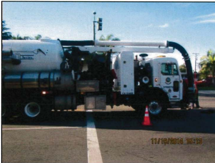
Photo 23: Crews securing area for mainline inspection
