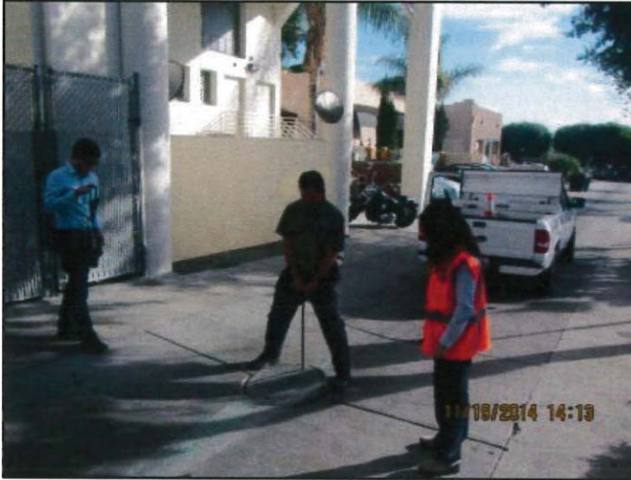
Photo 9: FOG sewer line inspection (view 1)
