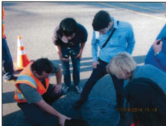
Photo 24: Mainline inspection with Miller
