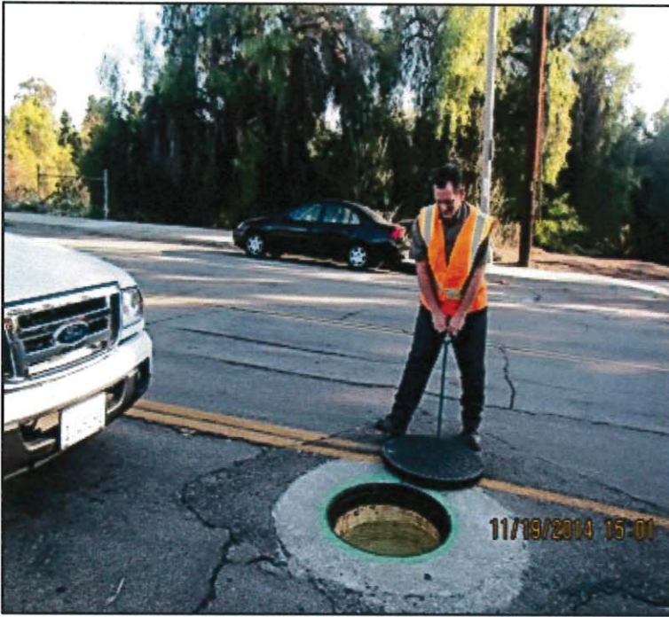
Photo 21: Miller opening rehabilitated manhole for inspection
