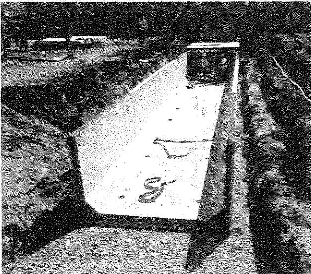
Fig. C-3: Installing precast concrete vault sections
