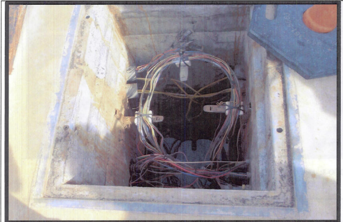
PHOTO 1: View of underground utility box which was inundated with floodwater. After entering the utility box, the floodwater then proceeded into the WWTP influent pump station through electrical conduits, causing the electrical failure and resulting sewer overflow.
