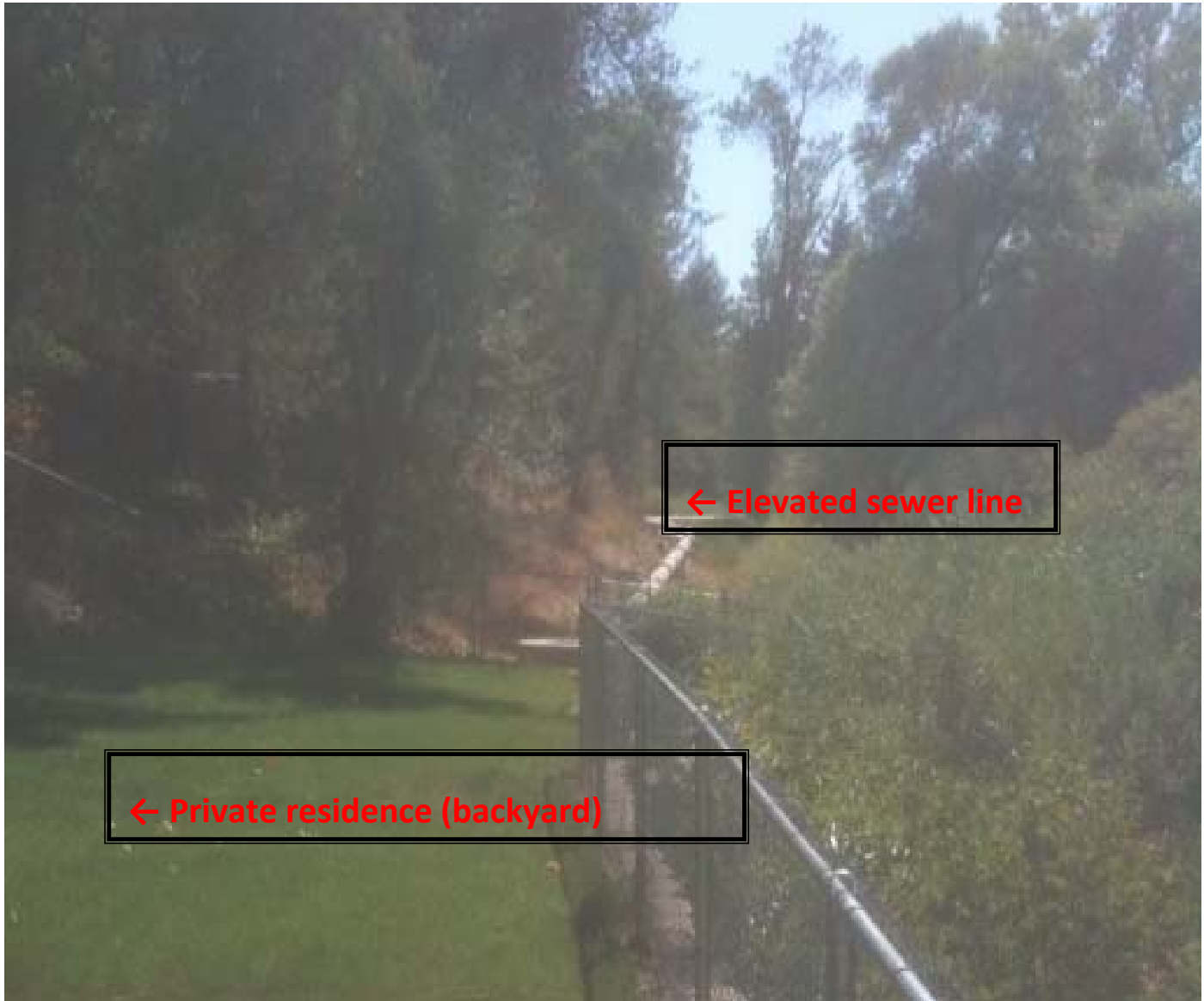
Photo 20: Jenny Creek elevated gravity sewer crossing
