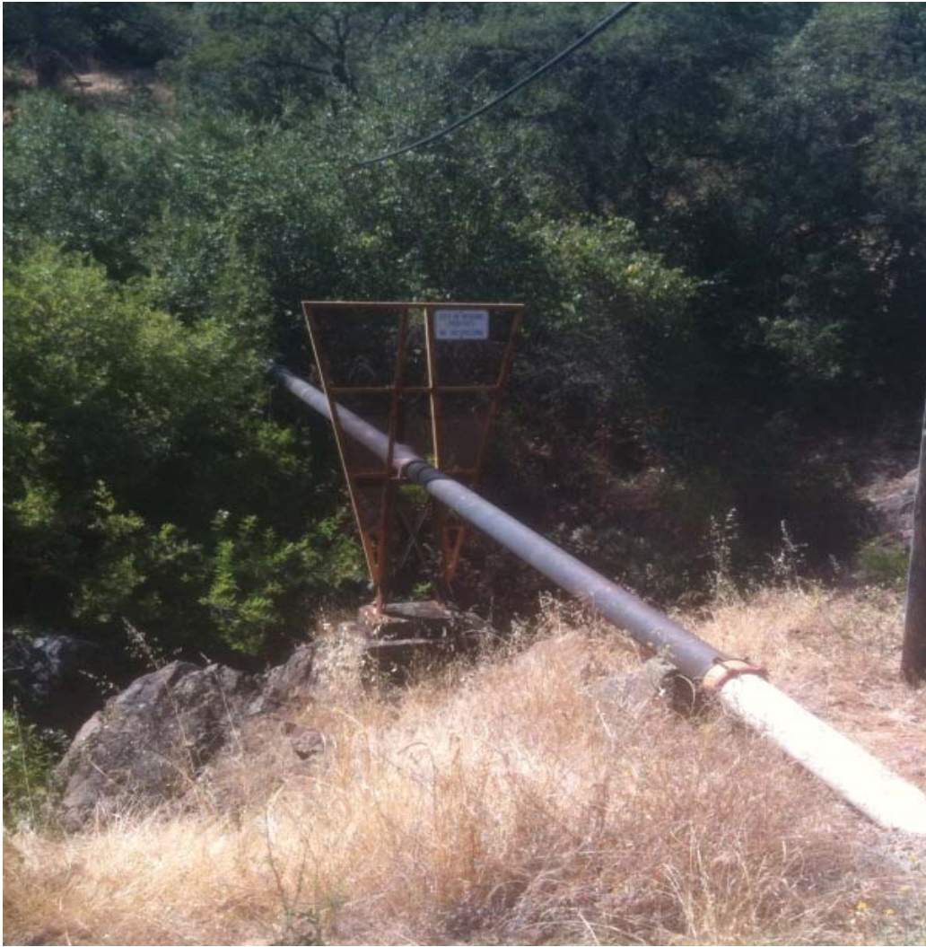
Photo 19: Jenny Creek elevated gravity sewer crossing
