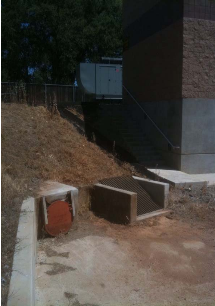
Photos 11-12: North Market lift station engineered impoundment gate valve and overflow drain (L), and impoundment levy (R)
