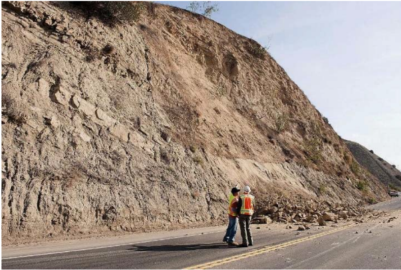
Figure C.26-1 Slopes Prone to Erosion and Sediment Discharge
