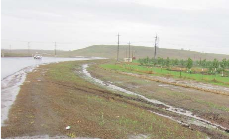
Shoulder graded; slope with netting and hydroseeding
