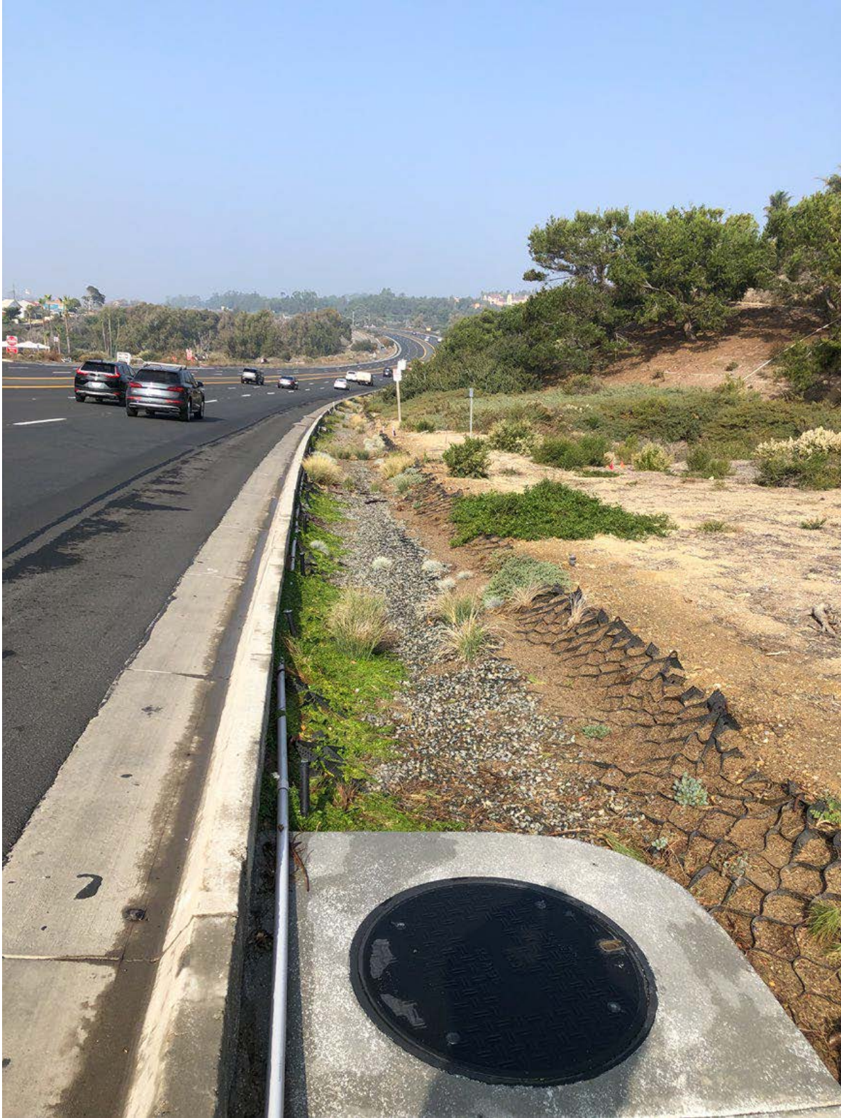
Figure E-8. After 12/09/21
