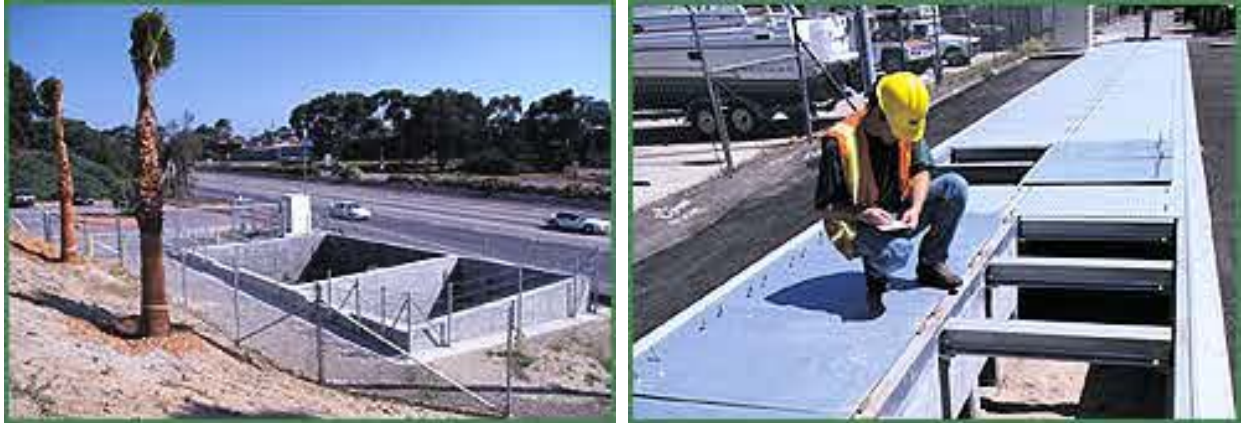
Figure D-5. Caltrans Media Filters (Austin Sand Filter [left], Delaware Sand Filter [right])
