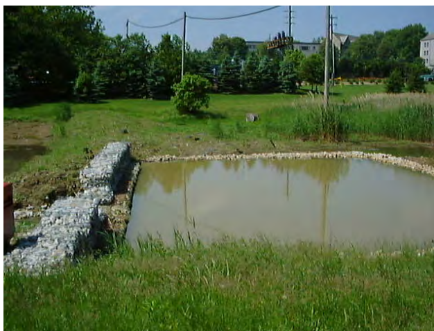
FIGURE 5-44 Villanova University sediment forebay. SOURCE: Reprinted, with permission, from VUSP. Copyright by VUSP.
