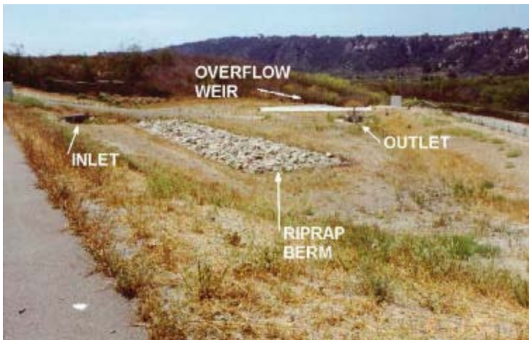
Figure 3-3 I-5/SR-56 Unlined Basin
