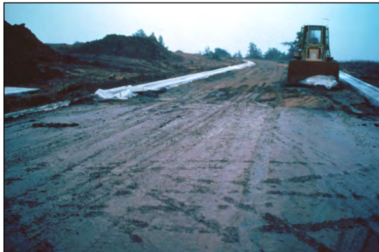
FIGURE 3-35 Construction site in early spring after snowmelt showing extensive sediment transport. SOURCE: Roger Bannerman, Wisconsin Department of Natural Resources.
