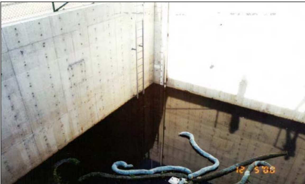
Figure 10-3 Internal View of an MCTT (Lakewood P&R)
