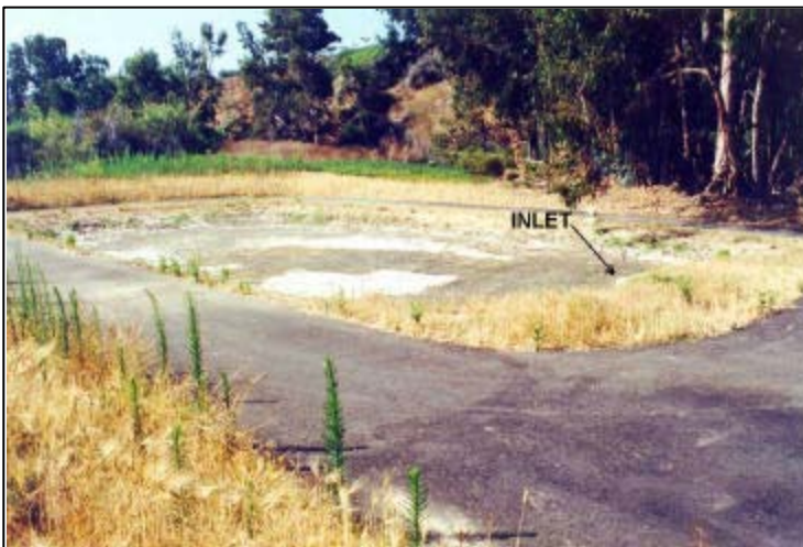
Figure 5-1 I-5/La Costa Infiltration Basin
