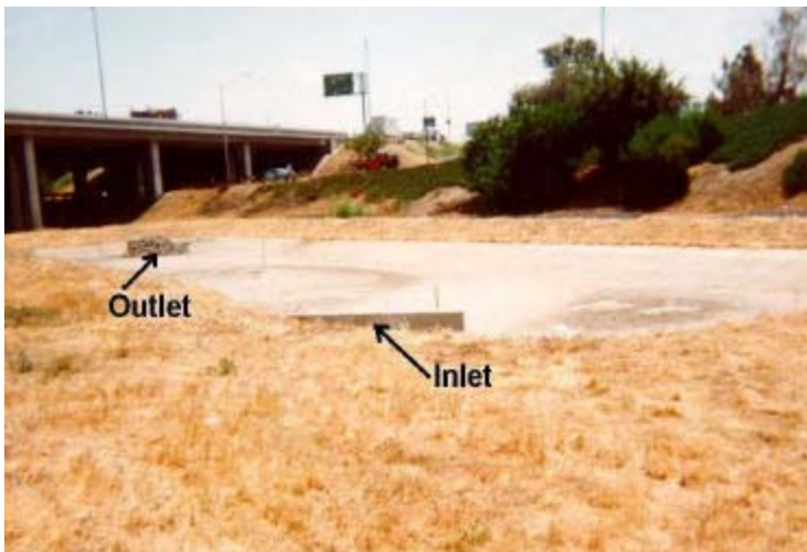
Figure 3-4 I-5/I-605 Concrete Lined Basin
