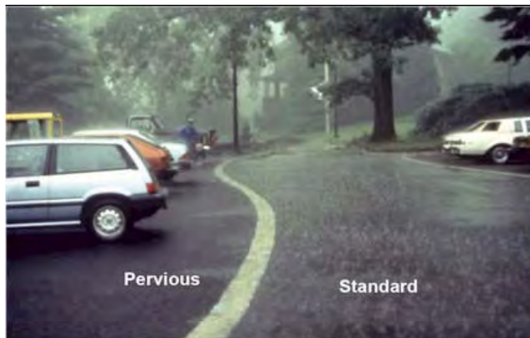
FIGURE 5-29 Porous asphalt. SOURCE: PaDEP (2006).
