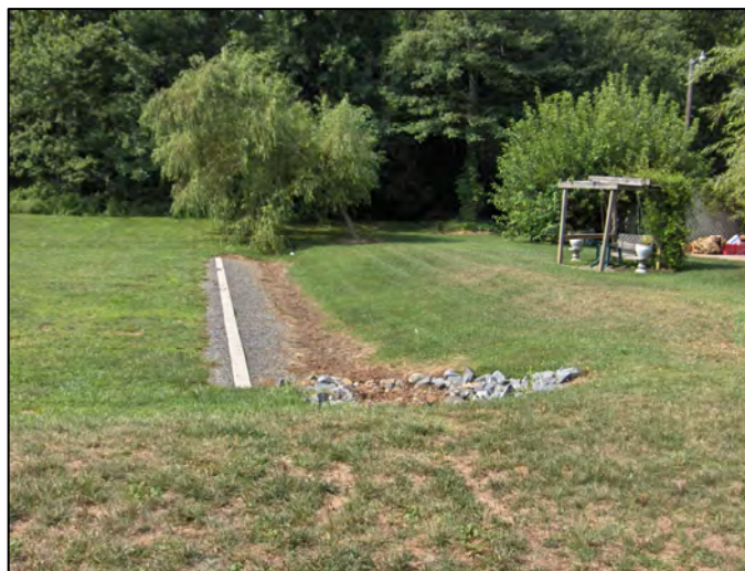
FIGURE 5-11 Level spreader. SOURCE: Robert Traver, Villanova University.
