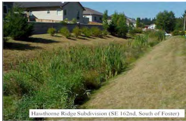
FIGURE 5-16 Vegetated swale. SOURCE: PaDEP (2006).
