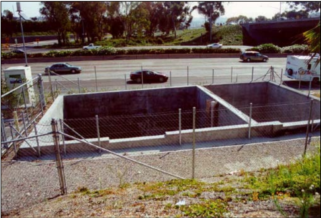
Figure 2-2 I-5/SR-78 Austin Sand Filter
