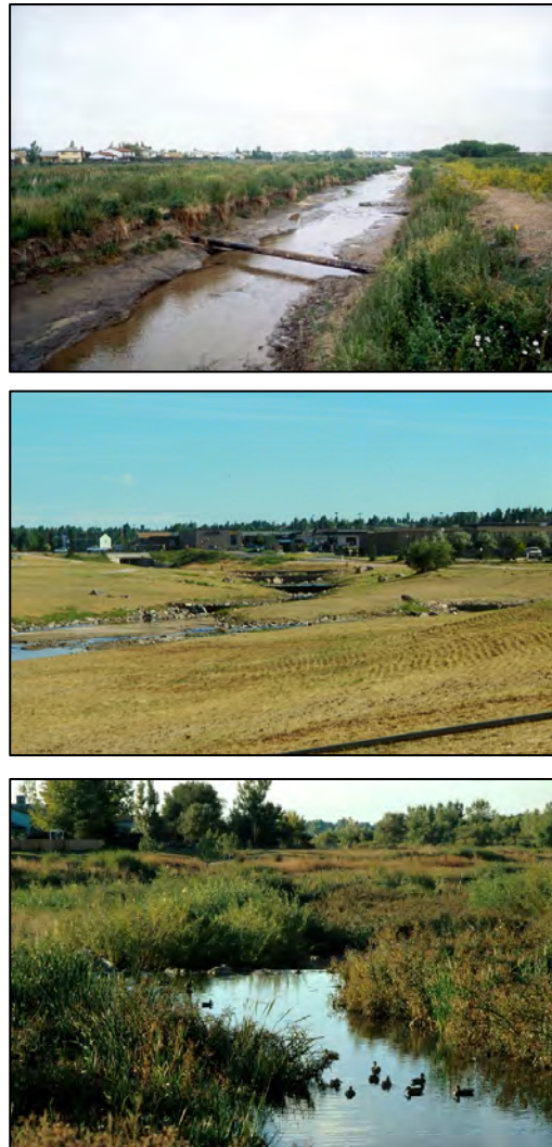
FIGURE 5-48 Three photographs illustrate stream rehabilitation in Denver. The top picture is a creek that has eroded in its bed due to urbanization. The middle picture shows a portion of the stabilized creek immediately after construction. Check structures, which keep the creek from cutting its bed, are visible in the middle distance. The bottom image shows the creek just upstream of one of the check structures two years after stabilization. The thickets of willows established themselves naturally. The only revegetation performed was to seed the area for erosion control. SOURCE: Courtesy of Wenk Associates.
