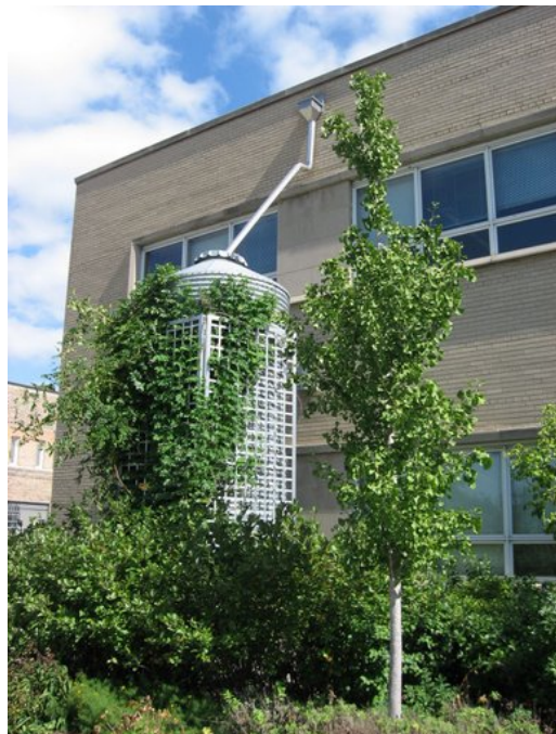
Figure 5. Rain water cistern.
