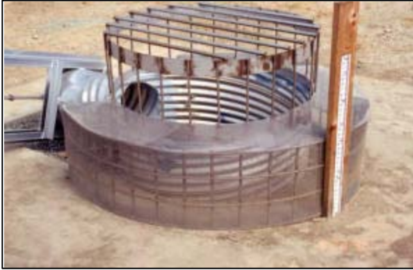
Figure 3-1 District 11 Outlet Riser
