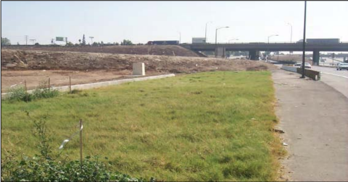
Figure 8-1 Biofiltration Strip (District 7, I-605/SR-91)
