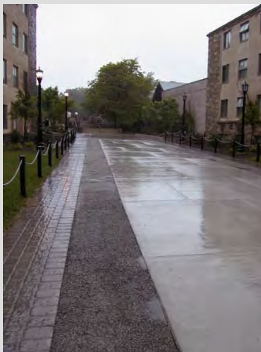
Note the runoff from impervious concrete spilling over to the pervious concrete. SOURCE: Robert Traver, Villanova University
