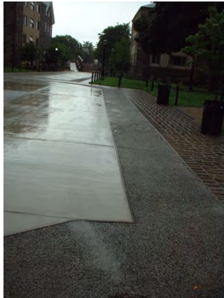
FIGURE 5-31 Pervious concrete at Villanova University. SOURCE: Reprinted, with permission from Villanova University. Copyright by VUSP.
