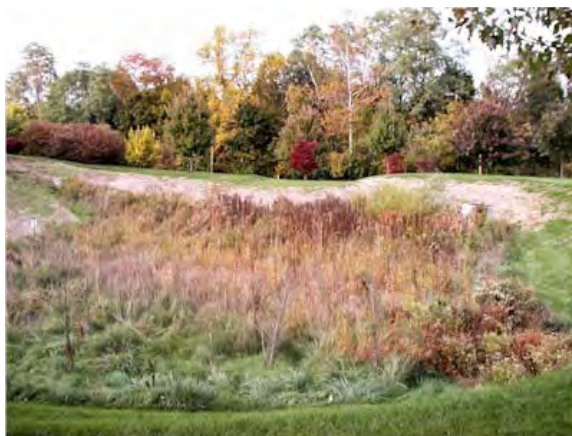
FIGURE 5-43 Dry extended detention pond. SOURCE: PaDEP (2006).
