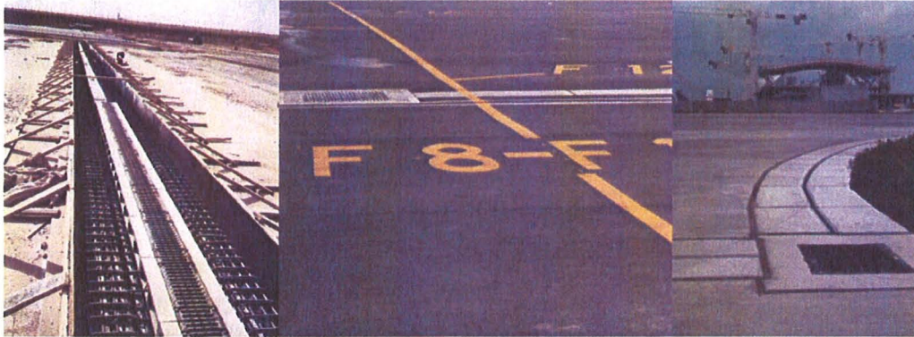
Safe airfield drainage per FAA Regulations excludes open ditches, trenches or non-frangible objects over 3 inches high.
