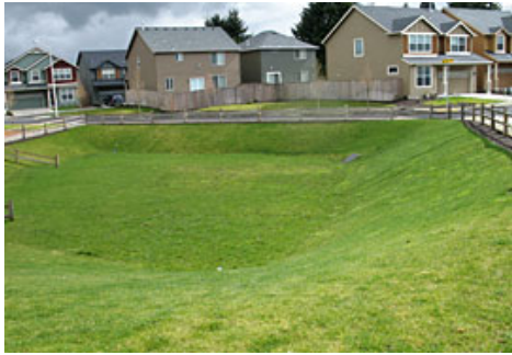
Figure 1. Detention basin (Stormwater Partners SW Washington)
