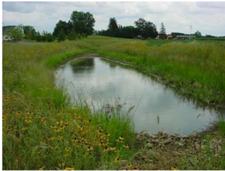
Figure 1. Wet pond (MN Pollution Control Agency)
