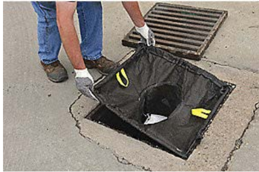
Figure 1. Drain inlet insert (Grainger)
