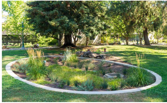
Figure 1. Bioretention planter
