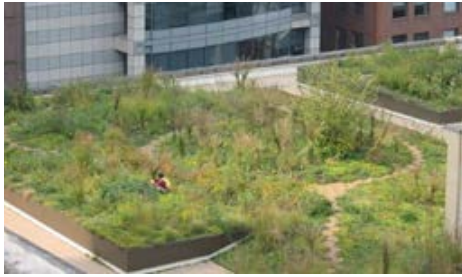
Figure 1. Green roof (Center for Neighborhood Technology)
