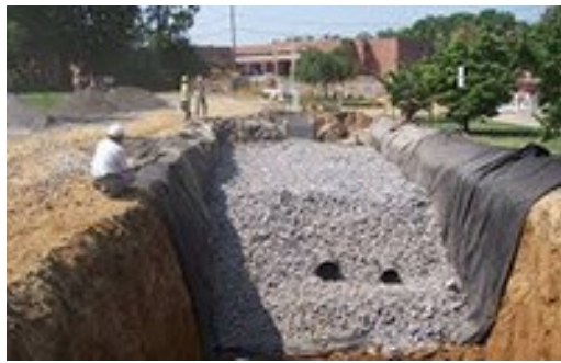
Figure 1. Infiltration trench (Richland Soil and Water Conservation)
