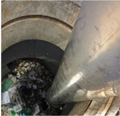
Figure 1. Hydrodynamic separator (EPA)
