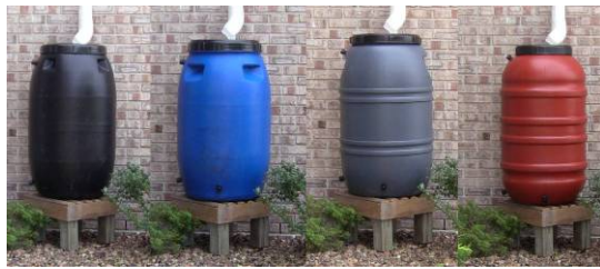
Figure 1. Aboveground storage (Porter County IN)
