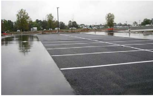
Figure 1. Porous pavement (EPA)
