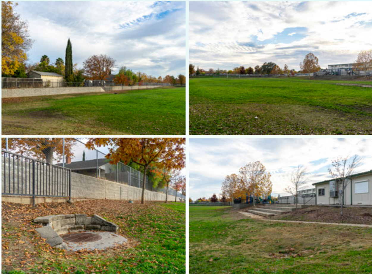
Figure VIII-2. Regional detention basin built with a soccer field at Leonardo Da Vinci Elementary School, Sacramento
