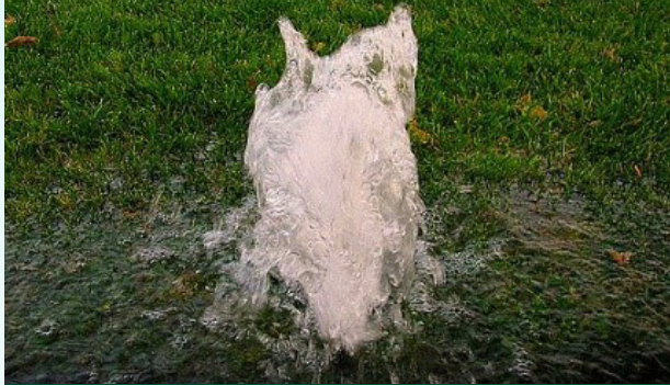
Flooding Due to Broken Sprinkler Head
