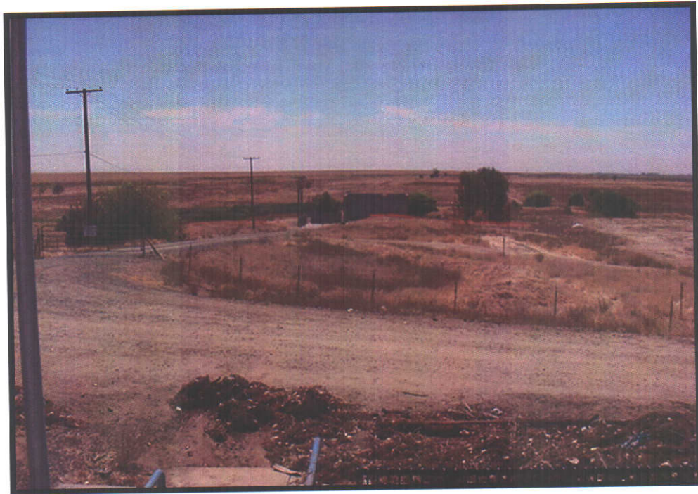
9. View downstream to Papazian Power Plant along the buried pipeline section of the Le Grand Canal.
