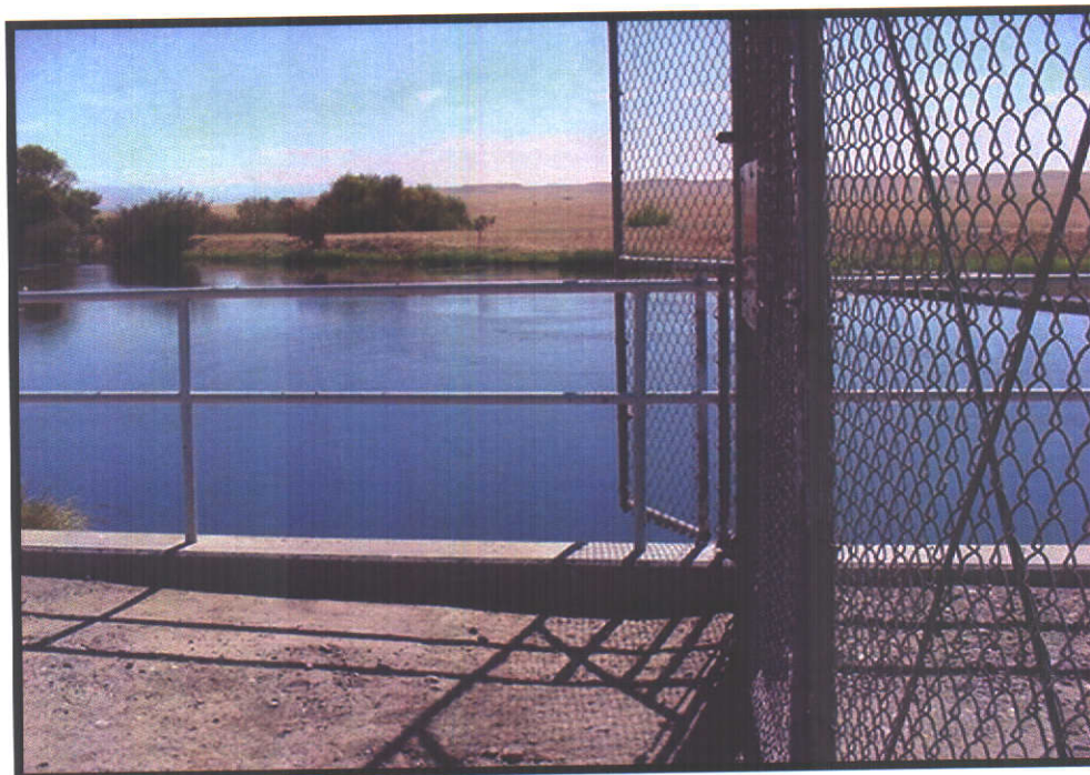
2. View upstream of Parker Power Plant, which shows the Main Canal.
