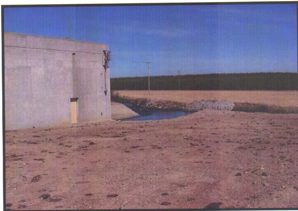
7. View downstream from Reta Power Plant.
