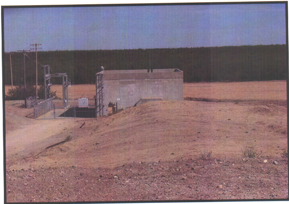
5. View downstream to Reta Power Plant on the Main Canal.
