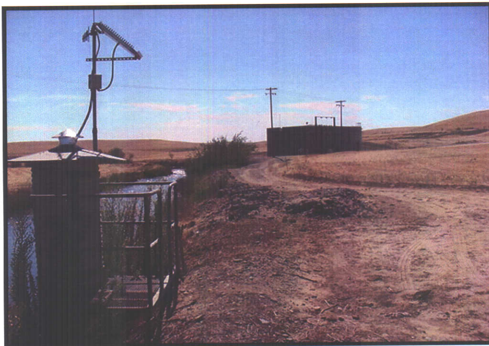
8. View upstream along the Main Canal toward Reta Power Plant.
