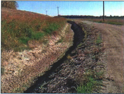
PHOTO 9 – Water Delivery Ditch.
