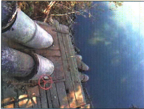
PHOTO 5 – Existing Grimes Diversion.
