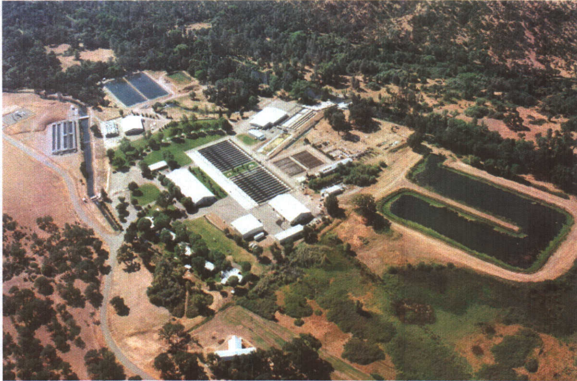
Location of water use (Coleman National Fish Hatchery)
