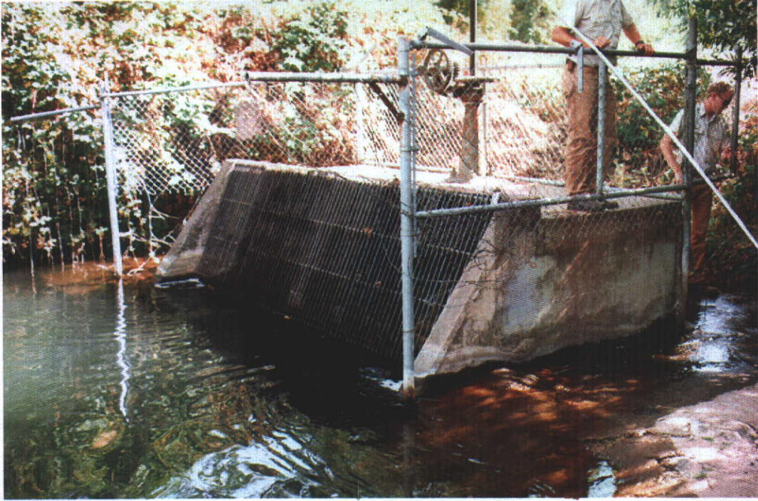
CNFH Intake 1 (on Coleman Powerhouse tailrace)
