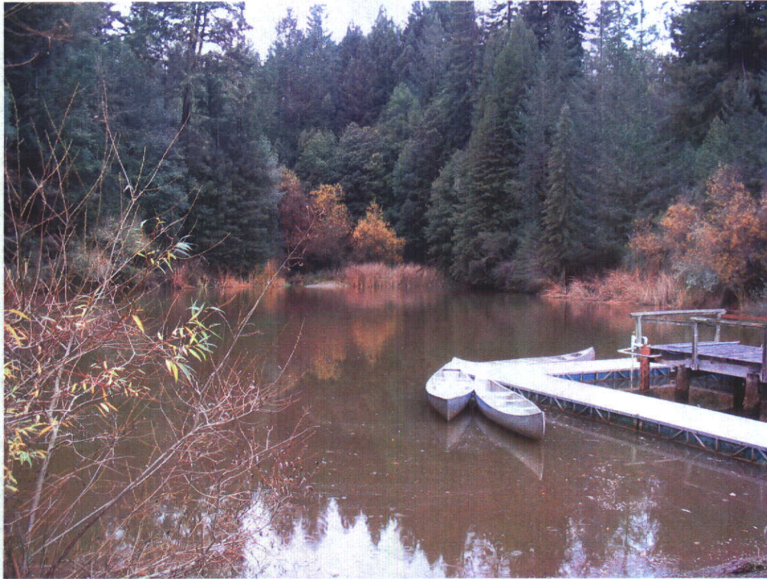
View of reservoir looking upstream from dam. Diversion piping can be seen at end of dock.
