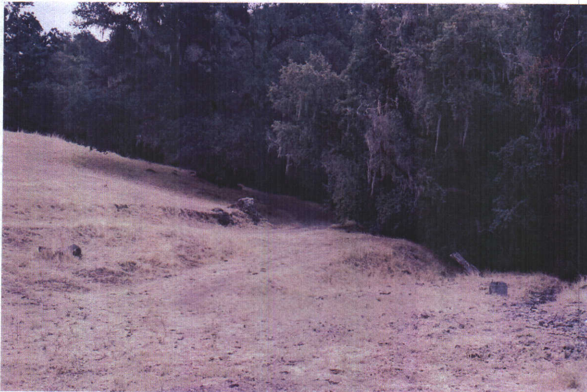
Photo looking northeast immediately upstream from the point of diversion (Reservoir B)
